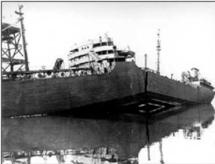
Fig. 10.1.2 Collapse of Liberty Ship T2 tanker "Schenectady"
