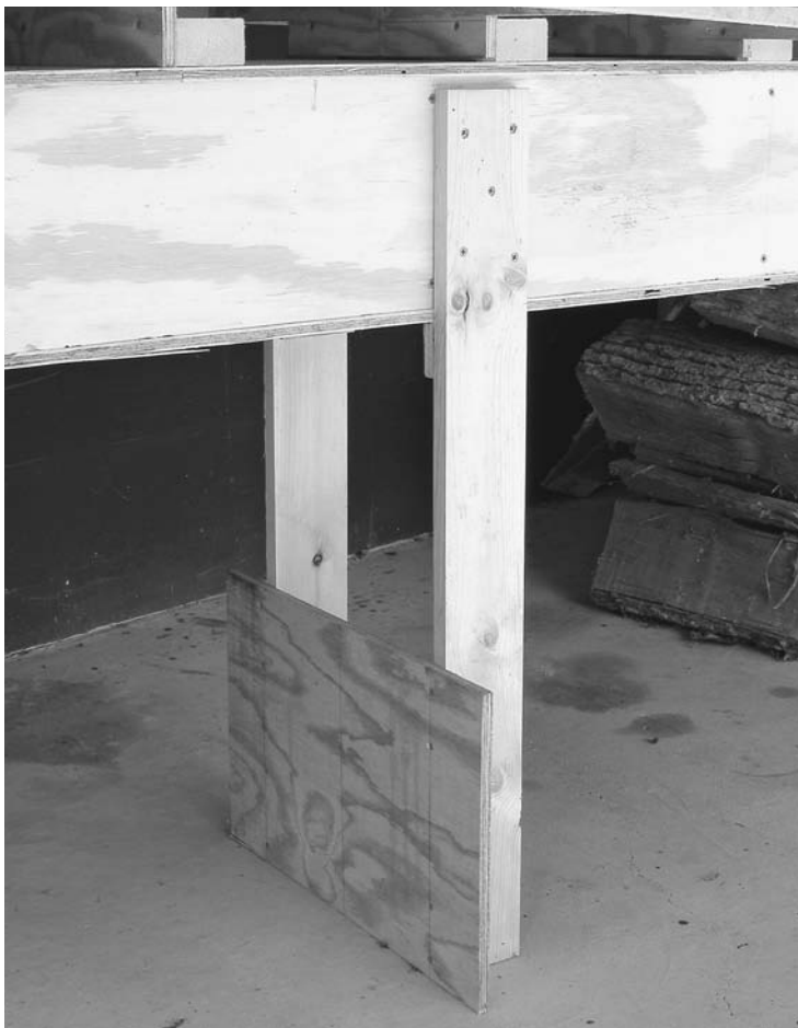
FIGURE 4.3. Strongback legs and foot.
