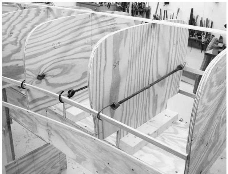
FIGURE 6.9. Bungee cords temporarily hold strips in place for attachment.
