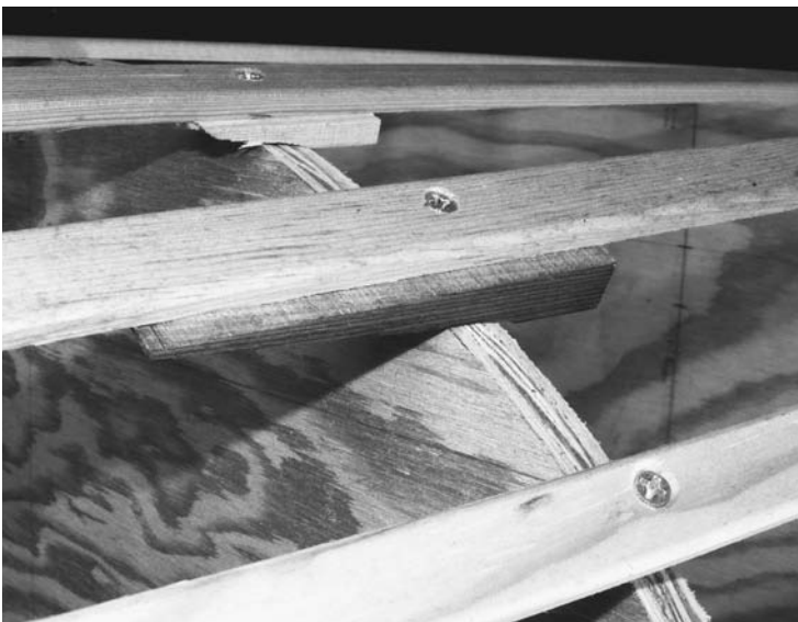
FIGURE 6.11. A wedge of wood can be placed between a station and a stringer to support the stringer into a smooth curve. Two of the stringers here have wedges.
