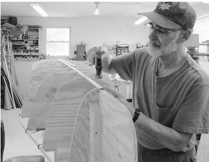
FIGURE 6.7. A temporary keel strip is tacked in place to hold the stations vertical.
