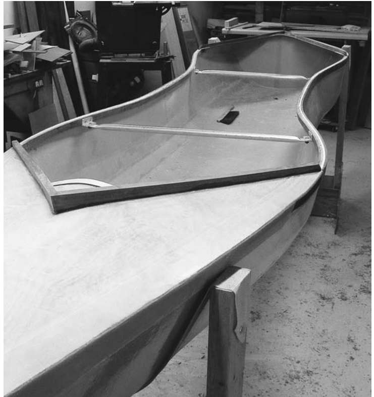
FIGURE 11.16. A deck with spray rails added.
