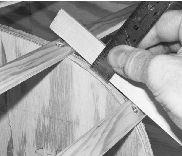
FIGURE 6.15. Measure the clearance between station curves and spans between stringers. The strips pictured are 2½ inches apart, and minimum clearance should be 0.09 or \frac{3}{32} inch. Where strips are farther apart, minimum clearance should be greater; \frac{1}{8} inch is good.
