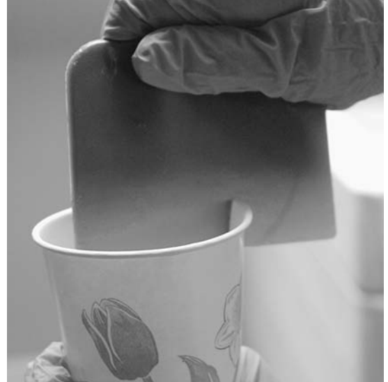
Figure 9-20. Remove excess epoxy on your squeegee with a grunge cup. Cut a slit at the top edge of the cup. Drag the squeegee through the slot to scrape off the resin. A paper cup works better than plastic because it does not rip as easily. I cut the slit through the doubled-up area of the paper where it is a little stronger. Don't use the gunk you scrape into the cup for anything; just let it harden and discard it.
