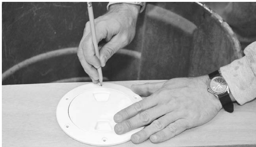
Figure 11-29. Install access ports into all the trapped-air spaces under the seats. This allows for inspection, lets you dry out any condensation that may arise, and provides convenient dry storage. Mark the large holes with a compass, then cut them out with a jigsaw. The mounting holes can be marked using the hatch as a jig.
