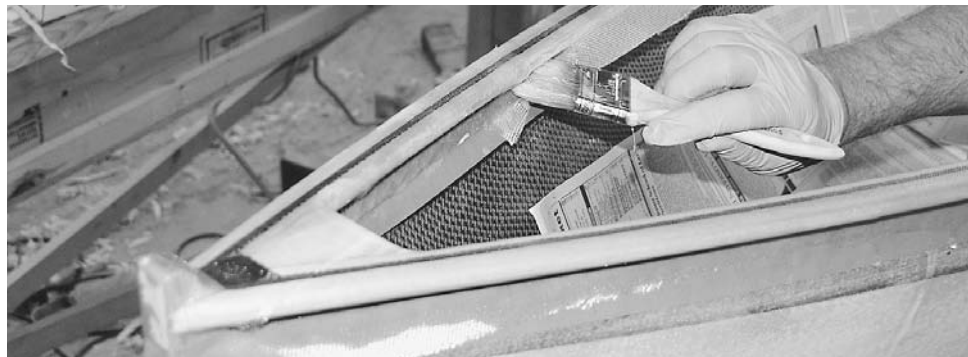
Figure 12-35. The gunwale will be covered with 3-inch-wide bias-cut strips of fiberglass. Run masking tape about \frac{1}{4} inch below the bottom of the gunwale, then lay out the glass strips.
