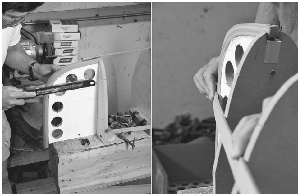
Figure 5-29. If you don't have a pattern for the bevel angle of the inner stem, you can bevel it while on the forms. Use a strip of wood laid over the forms to look for a tight fit flat against the side of the stem.
