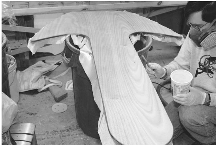
Figure 11-28. To protect the plywood against checking and rot, cover both the top and bottom surfaces of all the plywood parts with 4-ounce cloth. The cloth wraps down the radiused edges. When you flip over the parts to glass the other side, trim the glass flush and then overlap the edge with the new glass. Seal the end grain that will be assembled against the boat, just to be sure there is little chance for water to penetrate the plywood.
