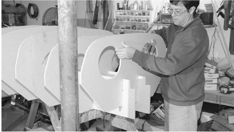
Figure 11-9. The simplest form of strongback is some plywood or, as in this case, particleboard slotted to accept the forms. This slotted beam works particularly well on a short boat where only one 8-foot length is required. Because of the size of the forms on the Coot, some large holes cut in the forms keep the weight down. Chesapeake Light Craft cut these forms for me with a CNC router, but they could be cut at home using a band saw or jigsaw. The slotted strongback has 1/2-inch-wide slots spaced every 12 inches.
