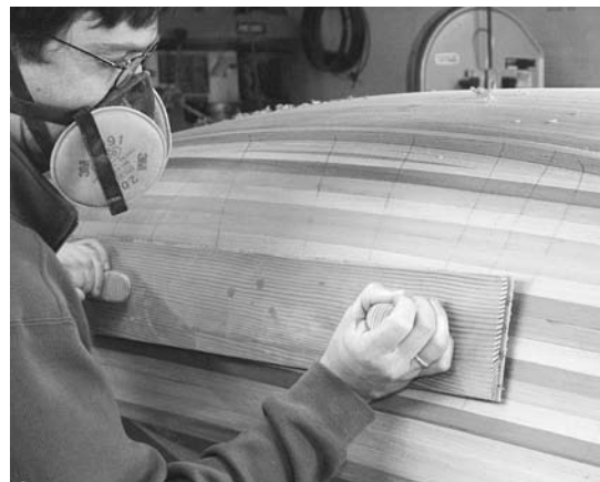
Figure 7-8. By working until all the pencil marks are gone you will be sure the whole surface has been sanded and is quite fair. This fairing process can be done with very coarse sandpaper such as 40- or 60-grit. Try to sand with the grain to minimize the scratches.
