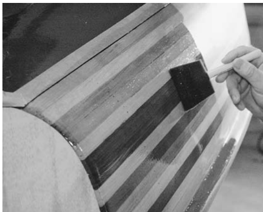
Figure 10-12. Finally, lightly tip off bubbles with quick, even strokes. Brush in one direction, from the drier side to the wetter. Lift up the brush while you are moving. Double-check for holidays as you work. As soon as you finish one section, move on to the next section. This is not a time to answer the phone or go eat cookies. Do the whole boat without stopping. When you are done, peel off the tape and leave the area so you don't stir up dust.
