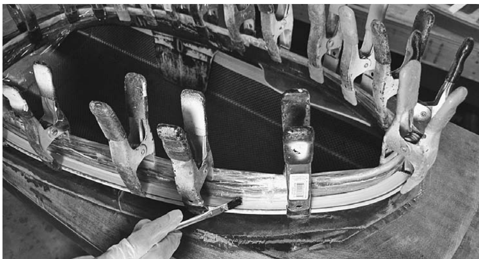
Figure 13-53. I usually finish the coaming at this time, but you could do these steps anytime after installing the riser. I use the coaming riser as a form to laminate the coaming lip. The strips should be about \frac{3}{16} to \frac{1}{4} inch wide and about \frac{1}{16} to \frac{1}{8} inch thick to make the bends. You will need enough strips to make a lip \frac{3}{4} to 1 inch wide. Wrap the coaming riser with tape or stretch wrap (either plastic food wrap or binding wrap available at office supply or woodworking stores) so the laminations do not end up glued in place yet. The strip length should be just short of long enough to go all the way around the cockpit.
