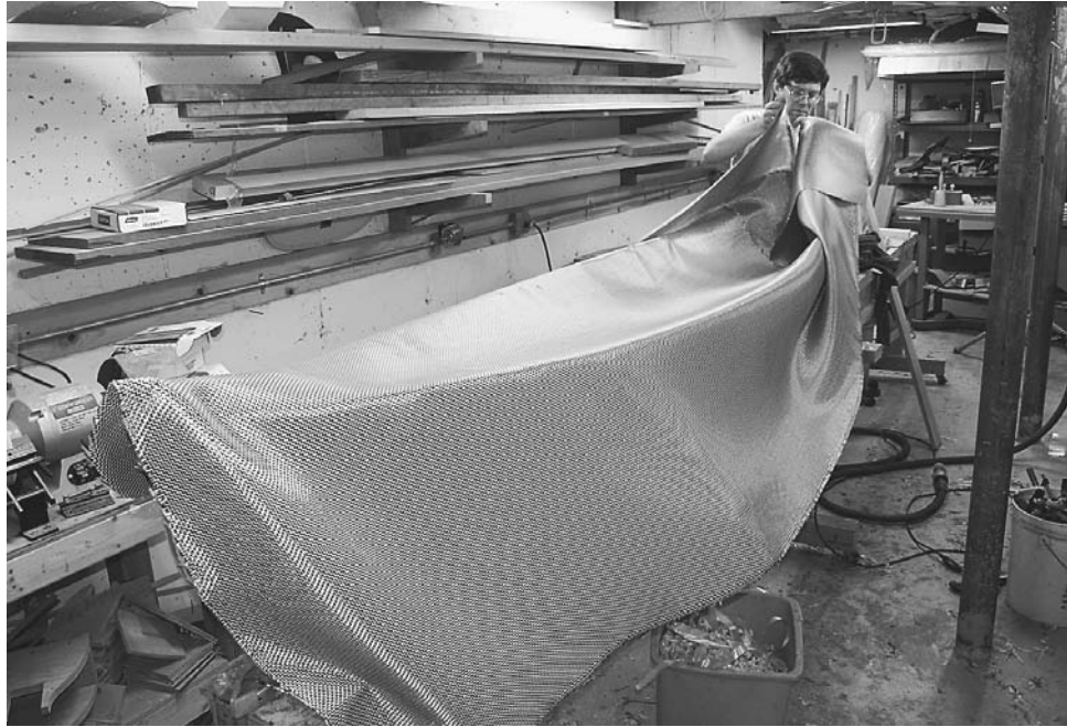
Figure 12-25. I used a hybrid carbon-Kevlar cloth on the inside. This weave has an evident pattern that will get distorted if the cloth is handled roughly. While not the end of the world structurally, distortions will be noticeable in the finished product.
