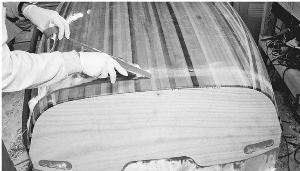
Figure 11-24. After the epoxy has stiffened up a bit, but before it is really hard (1 to 2 hours after wetting out), trim off the excess glass right next to the masking tape. Use a light touch so you are not cutting into the older, harder epoxy and glass. Install a brand-new blade in the knife so it won't take much pressure to cut through the fresh glass and green epoxy. Peel off the tape as you go. If you see the tape pulling any uncut strands of cloth, cut them with the knife. The result is a smooth, clean line instead of the ragged edge.
