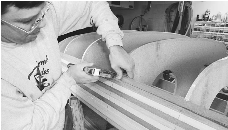
Figure 6-13. Staples provide by far the easiest and quickest method to temporarily clamp the strips in place while the glue dries. Press the joint close together and shoot a staple through the strip into the form. Rocking cove-and-bead strips a little bit as you press them in place will help seat them and spread the glue inside the joint. Keep stripping up the side until the strips start having to bend the "hard" way, across their width. On the last strip installed on the side, plane off the cove so it will be easier to shape the strips joining it later.
