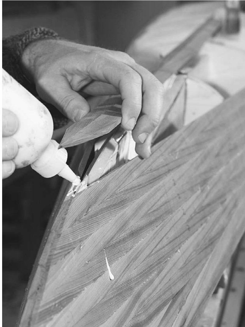
Figure 13-27. The change from strips running parallel to the side to strips running parallel to the centerline is always a little tricky. Here I have two strips running down either side of the centerline. These strips both need to be beveled to form a tight joint. At the ends the bevel will be quite severe because the strips will twist to meet the strips on the sides. After the bevel has been fine-tuned, the ends need to be tapered to fit against the existing strips. The two strips are held tightly together with masking tape. I put the tape in place while the strips were lying flat relative to each other. When I bend the ends of the strips down to install them in place, the tape will pull them together even tighter. These strips will have a lot of stress in them, so you will need to clamp them in place after gluing them down.
