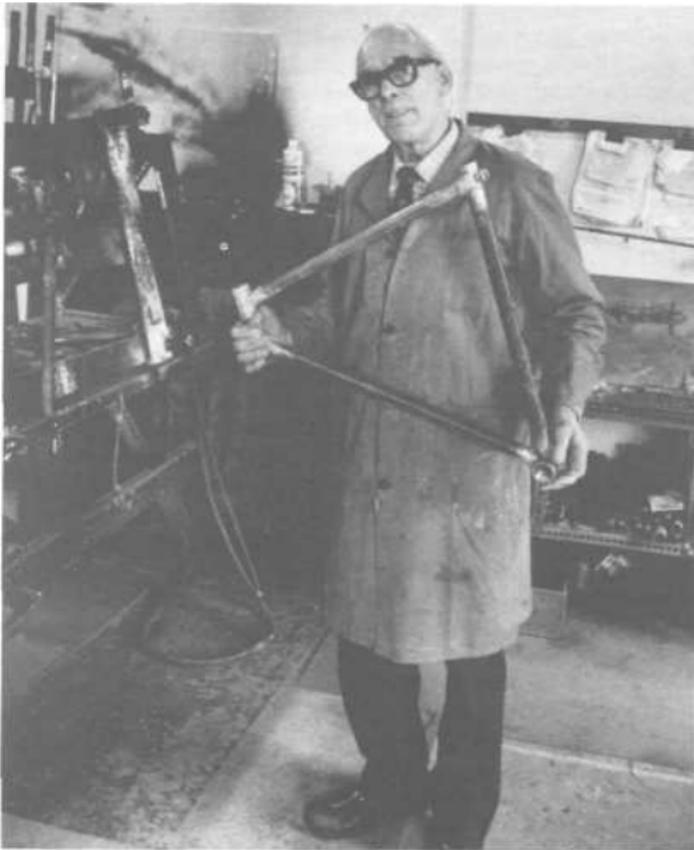
**Figure 7-1:** Harry Quinn with a complete main triangle of frame. The jig for brazing is on Harry's right.
