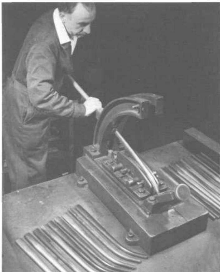
**Figure 2-4:** No machine has been developed to bend fork blades with more accuracy and care than this workman. All fork blades are raked by hand!
