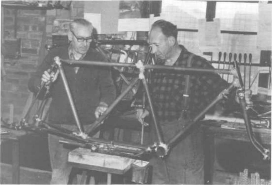
Figure 8-1: Jack (left) and Norman Taylor inspect a newly brazed tandem frame.
