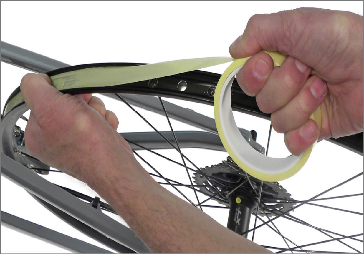
FIGURE 2.58: Install rim-sealing tape directly over valve hole
