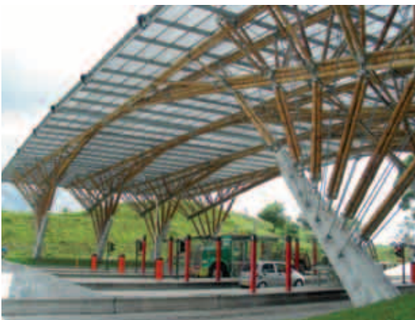
Figure 3-15: Bamboo as compression element in combination with steel as connector and tension wire
