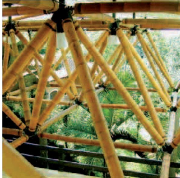
Figure 3-14: Bamboo space structure by architect Leiko Motomura (source: Amima)
