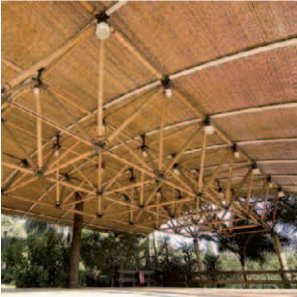
Figure 3-14: Bamboo space structure by architect Leiko Motomura (source: Amima)
