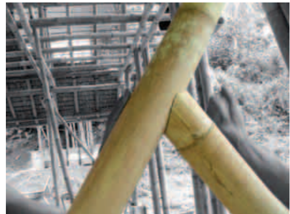
Figure 4-4: Fish-mouth joint, bamboo at the right side belongs to Group 1, but at the left side belongs to Group 5
