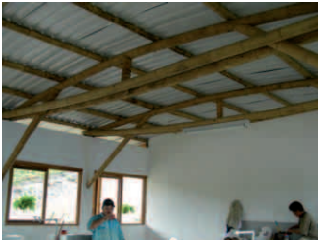
Figure 2-3 (above): Curve bamboos as roof frame
