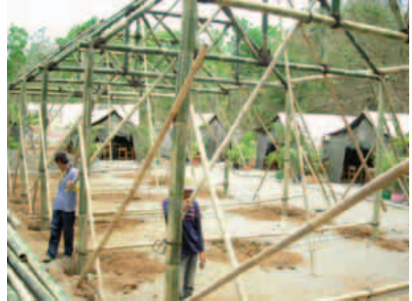
Figure 3-5: Planar frame in common vernacular bamboo construction (courtesy of AMURT)
