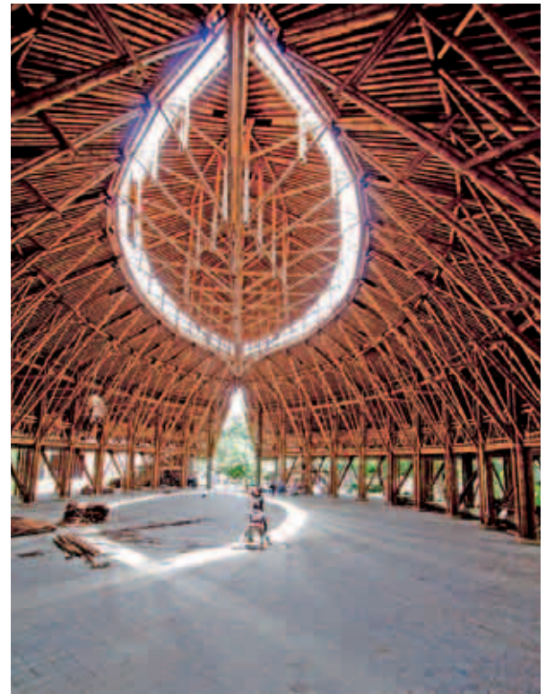
Figure 3-11: Three-dimensional frame and the beauty of the rhythm of repetitive frame in the Great Hall OBI by architect Andry Widyowijatnoko (courtesy of Eko Purwono)
