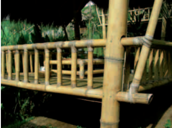
Figure 3-4: Traditional bamboo gazebo in Indonesia with positive fitting and lashing joint
