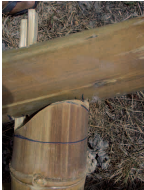
Figure 3-3: Fish-mouth joint with two pinned flanges (courtesy of Benjamin Brown)
