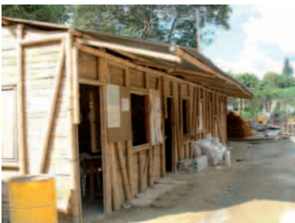
Figure 3-6: One layer frame of wall construction in Colombia (source: anonymous)
