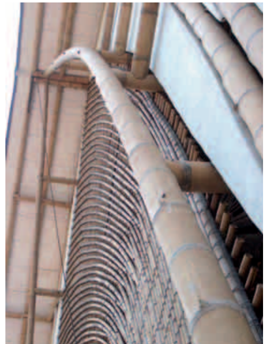
Figure 2-3 (above): Curve bamboos as roof frame
