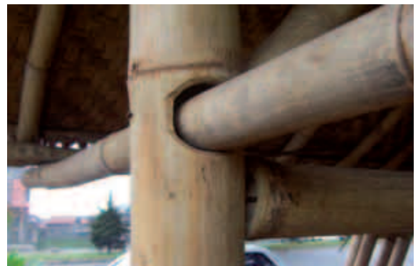
Figure 2-6: Positive fitting joint in an easy made temporary bamboo structure
