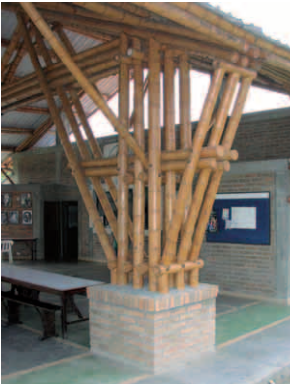
Figure 3-10: Two-dimensional frame with many layers (courtesy of Jörg Stamm)
