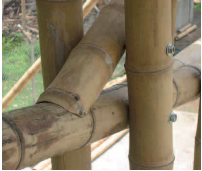
Figure 3-9: Eccentricity of load transfer in a joint (courtesy of Jörg Stamm)
