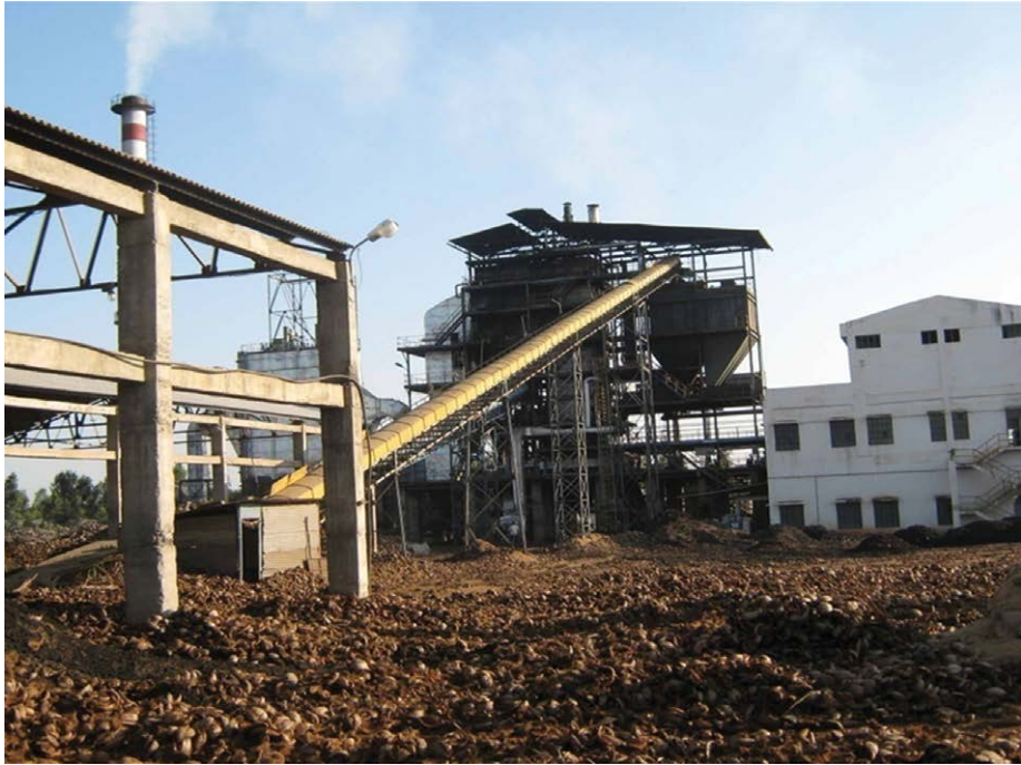
Fig. 2.24. A bamboo biomass power plant in India (Barathi, 2013).
