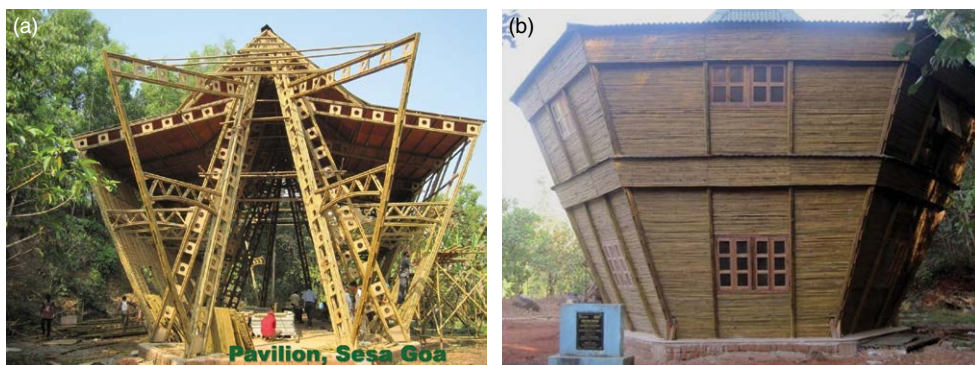
Fig. 2.110a,b. A bamboo pavilion (a) under construction and (b) after the completion of construction in Goa, India (KONBAC, 2013).
