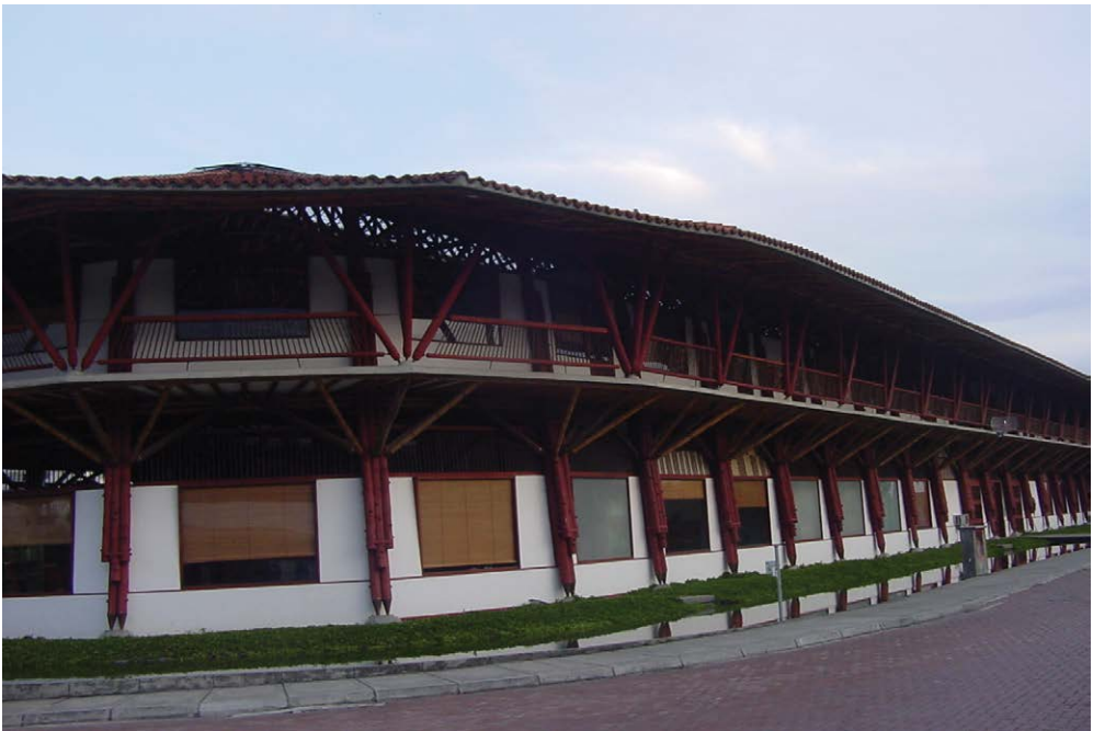
Fig. 2.64. The office building of Colombia's Ministry of Environment, which is mainly made of bamboo (Zhu Zhaohua).
