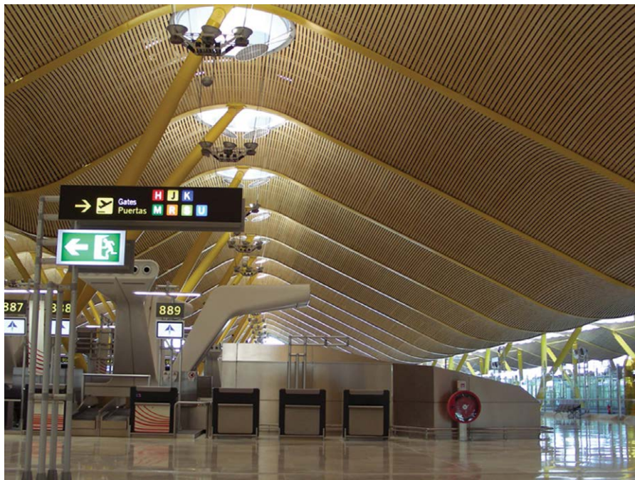
Fig. 3.123. Madrid Barajas International Airport in Spain showing the bamboo ceiling made of planks of multi-layered Moso bamboo veneer (photo by Dasso).
