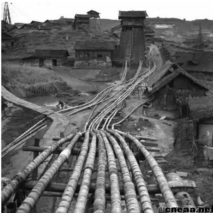
Fig. 2.61. Gas transfer using bamboo pipes (from the Museum of Salt Exploration in Zigong, Sichuan Province, China).
