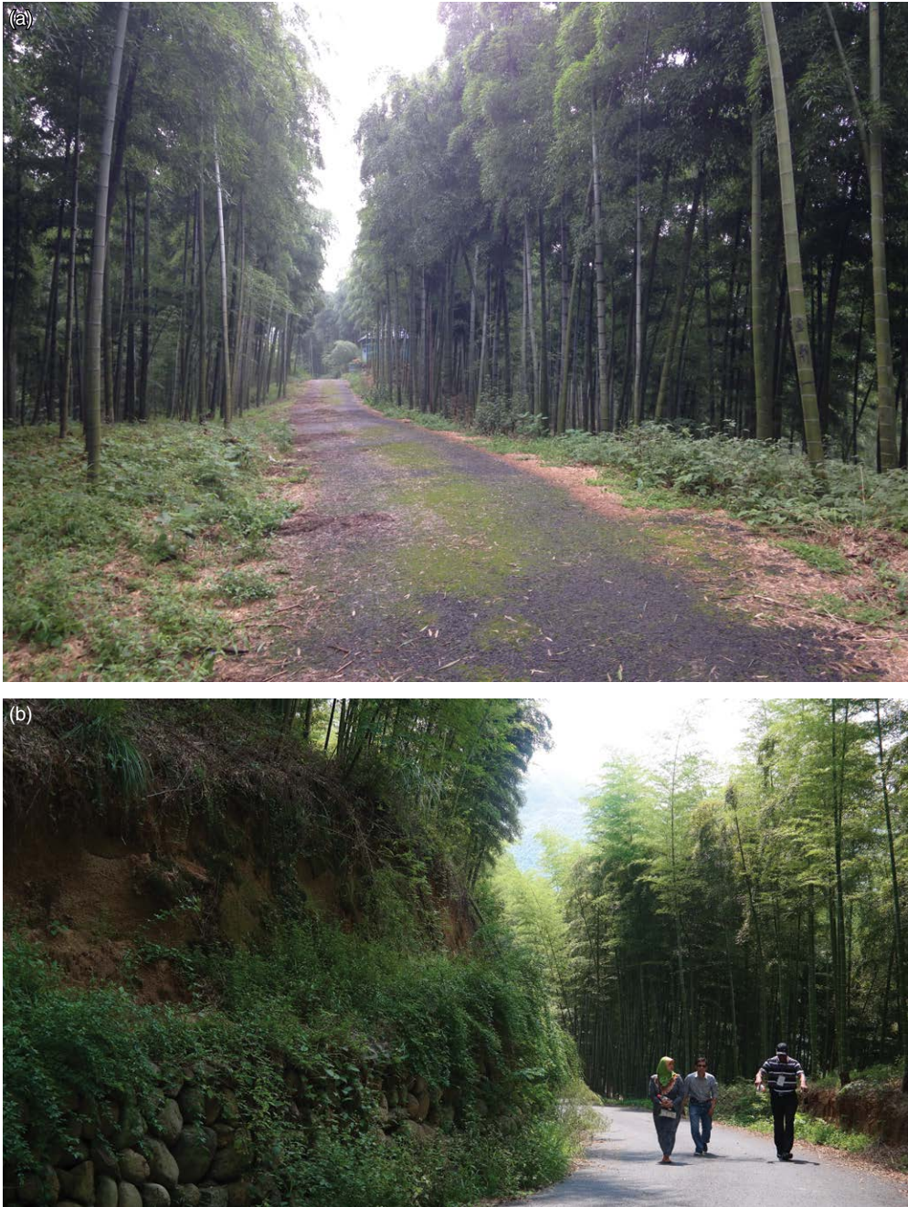
Fig. 3.76a,b. Photos of bamboo-lined forest road in Anji, Zhejiang Province, China (Zhu Zhaohua).
