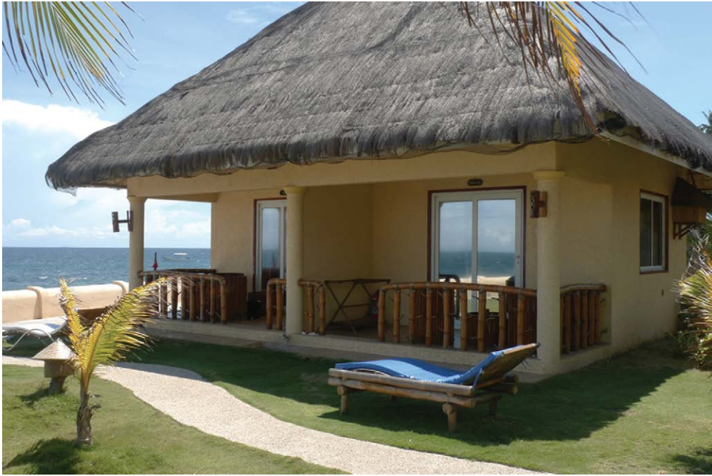
Fig. 3.89. A bamboo hotel on the beach by the sea in the Philippines (Zhu Zhaohua).
