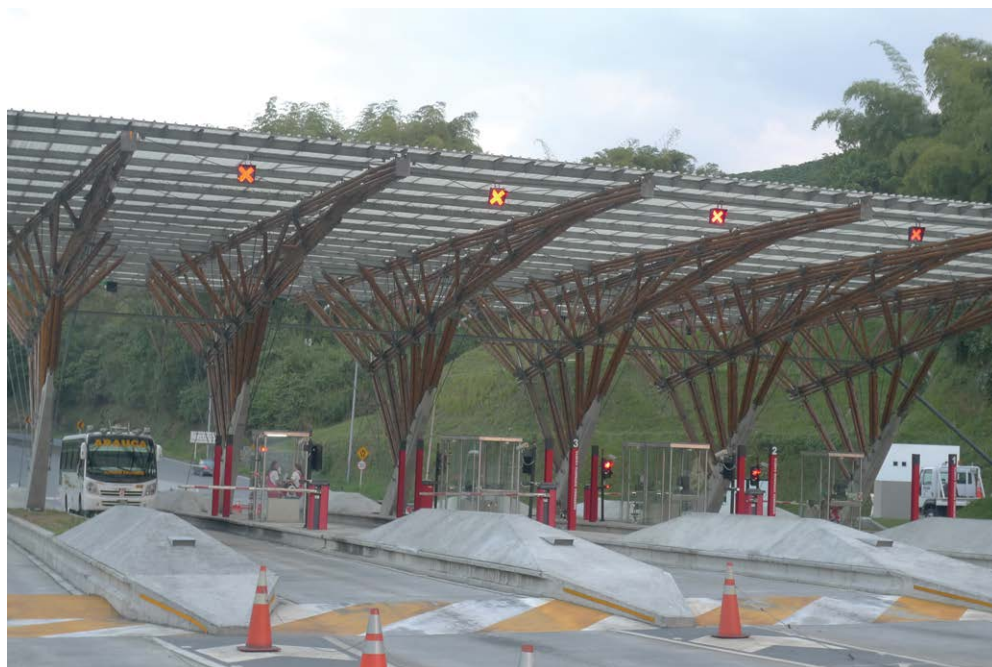
Fig. 3.97. A highway toll station made of bamboo in Colombia (Zhu Zhaohua).
