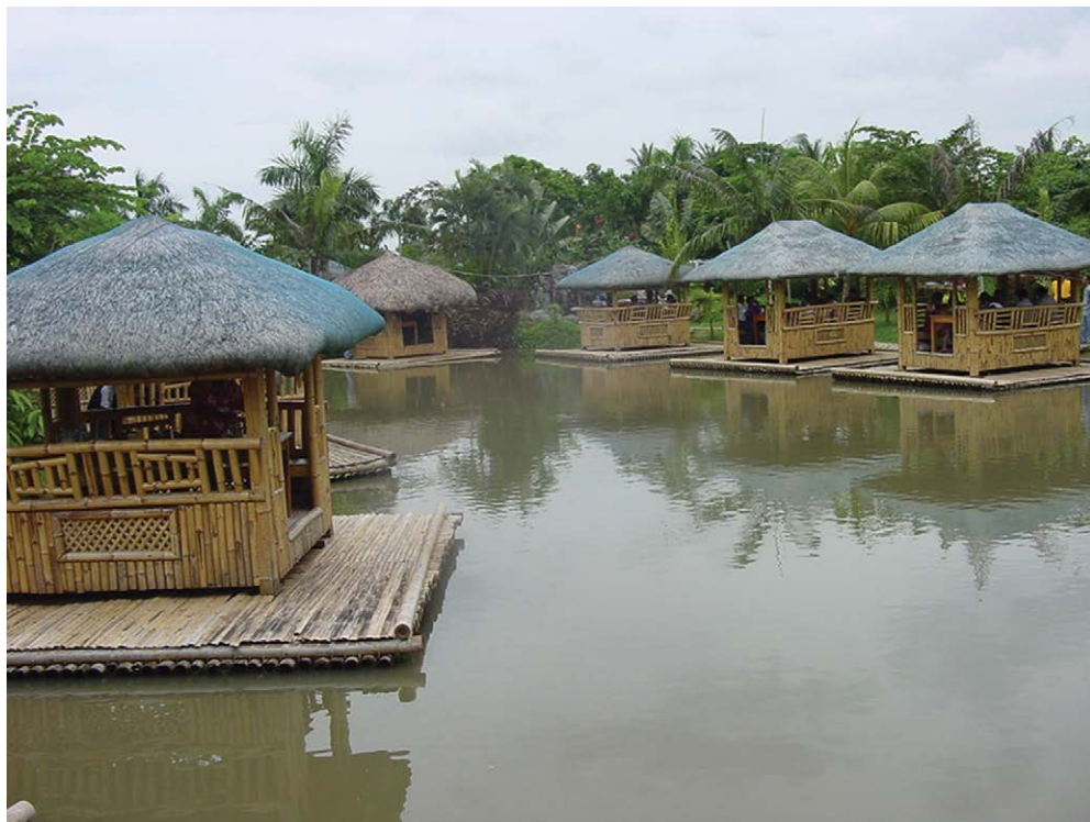
Fig. 3.48. A floating restaurant constructed of bamboo in the Philippines (Zhu Zhaohua).
