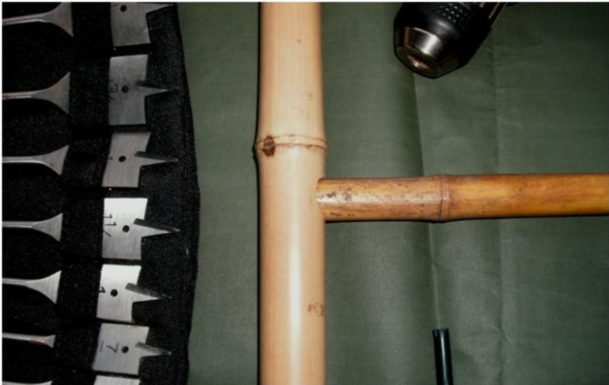
The cross-pole is then fitted snugly into the socket, until it touches the back wall of the upright.
