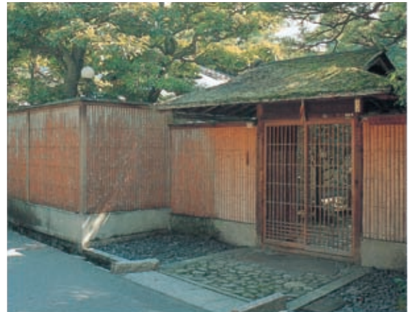
top Tokusa wall with changing heights separated by log posts
