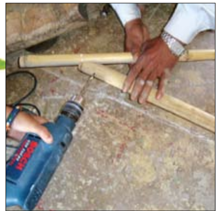
Drilling into Bamboo
