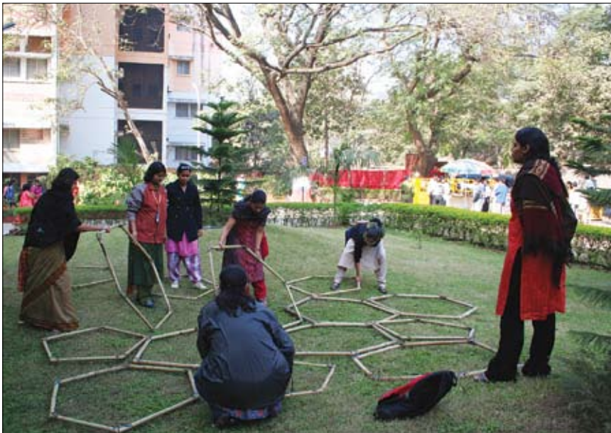
Hands –on experience: Students of M.Arch Environmental Science working with bamboo for constructing a geodesic dome.
