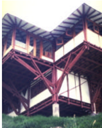
In the trusses at the base, the wooden poles are joined in the same manner as the roof bamboos.
