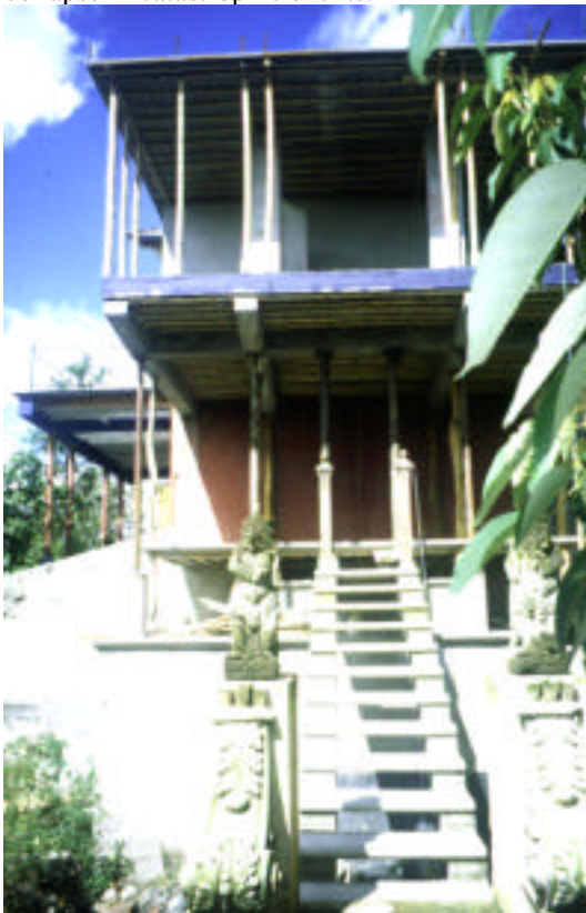
Velez' new office under construction
