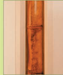
Bamboo in Adobe wall
