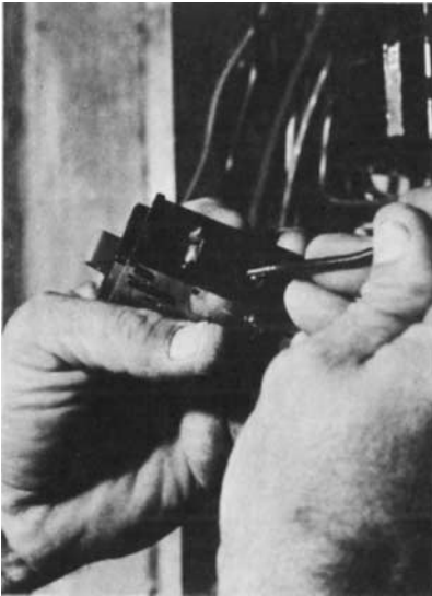
Figure 10-12 The black wire is attached to the dark screw of the circuit breaker. White (neutral) and bare, or green, insulated ground wires are ordinarily attached to the common grounding bar.
