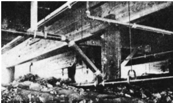
Fig. 14-27 Note the neat method of hanging pipe.
