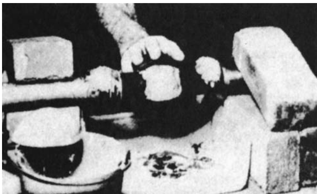
Fig. 10-7 A handy method of retaining under adverse conditions by building up the solder a little way from each side of the joint to be lifted off after completion.
