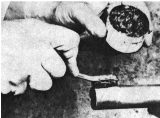
Fig. 12-14 Fluxing tube end. (Courtesy Copper Development Association)
