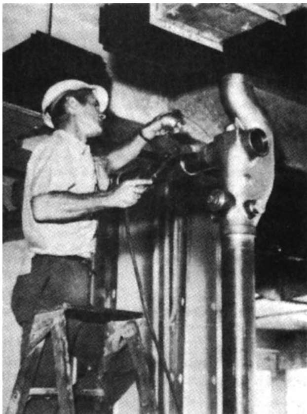
Fig. 15-15 Installing a copper Sovent system.
