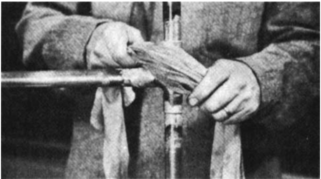
Fig. 12-9 Swabbing. (Courtesy Copper Development Association)
