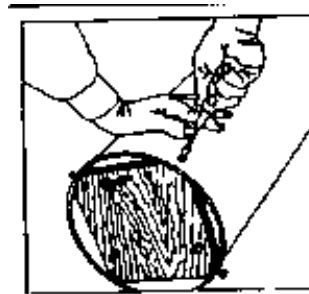
Screwing in the tailgate at all four corners. (Check the fit of the tailgate before installing the mirror).
