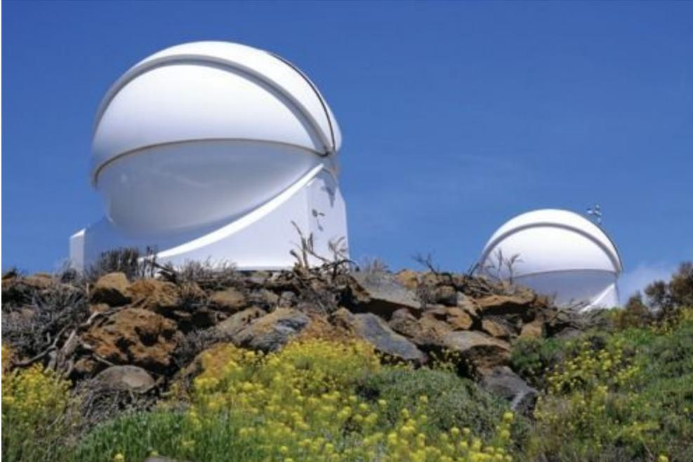
**Figure 1** The COAST dome on Tenerife. This houses the 14-inch telescope that you will use in this course, requesting images remotely. The dome visible in the background houses PIRATE (the Physics Innovations Robotic Astronomical Telescope Explorer), another Open University telescope. Behind this second dome can be seen the top of the mast holding the all-sky camera and a number of other weather sensors and instruments.
