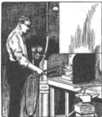
Melting a small quantity of platinum.
