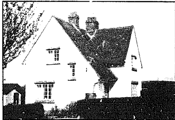
Chalk cement block house at Amesbury.
