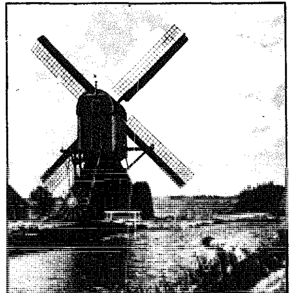
Fig 13. Traditional Windmills. (Upper left) Great Chishill post-mill, Cambridgeshire, oriented by a fantail. (Lower left) Chesterton tower-mill: 19th century photograph of a unique structure, possibly designed by Inigo Jones: oriented by a winch inside the cap. (Below) Dutch 'Waterwipmolen': a drainage post-mill oriented by a capstan wheel. (Top right) 'Tjasker', smallest and simplest type of Dutch drainage mill lifting water by means of an Archimedian screw. (Lower right) A 'paltrok', a uniquely Dutch type, designed for sawing wood. The entire structure rotated on rollers on a brick base. (Far right) The most characteristic Dutch type, a thatched smock-mill oriented from the outside by a capstan wheel and spars attached to the cap.
