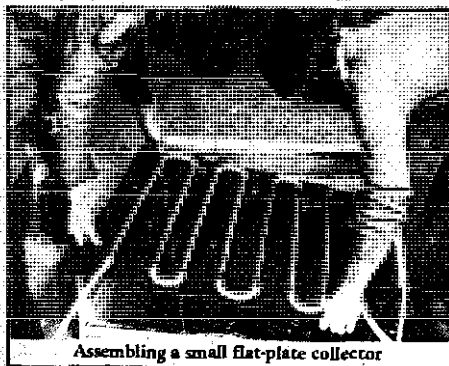
Assembling a small flat-plate collector
