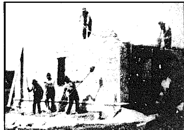
From the top: Adobe block production. Fine example of Devonian cob farmhouse, Budleigh Salterton. Cob building at Amesbury.
