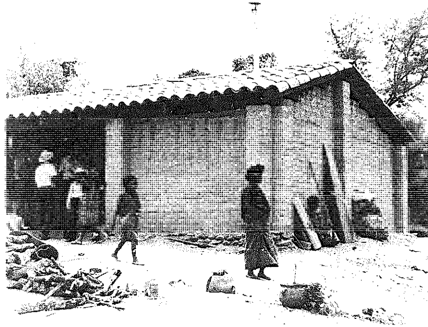
Fig. 6. First House Constructed by a Group of Three Families
