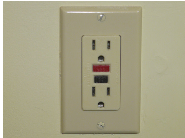
FIGURE 31-28 ■ A ground fault circuit interrupter electrical outlet with integrated test (black) and reset (red) buttons.
