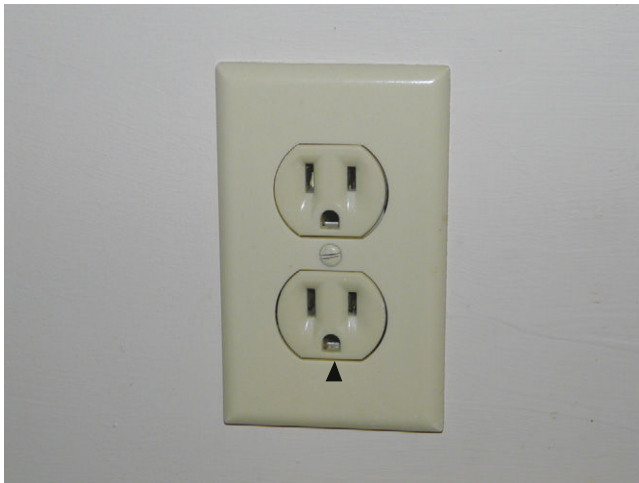
FIGURE 31-11 ■ Modern electrical outlet in which the ground wire is present. The arrowhead points to the part of the receptacle where the ground wire connects.
