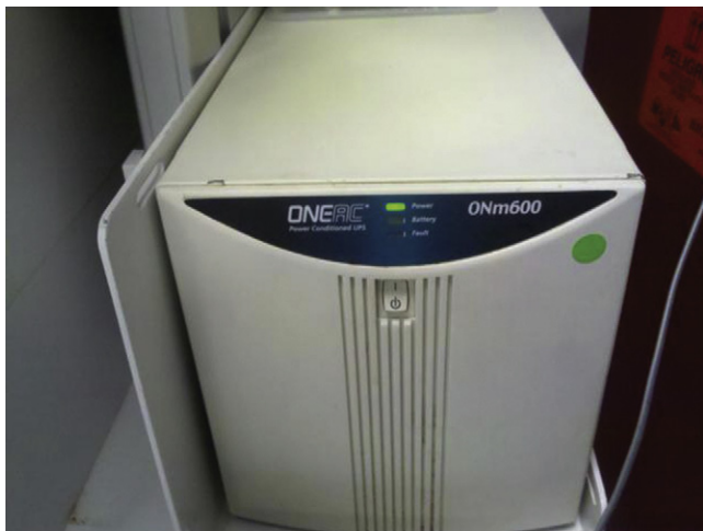
FIGURE 2-56 ■ Uninterruptible power supply unit supplements the workstation backup battery by energizing monitors and automated anesthesia record-keeping systems.
