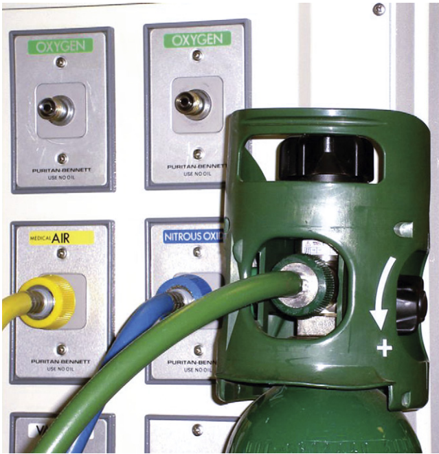
FIGURE 2-12 ■ If the wall oxygen supply fails, the machine's oxygen hose can be disconnected from the wall and reconnected to the 50 psig diameter index safety system connector on the oxygen tank shown in Figure 2-11.
