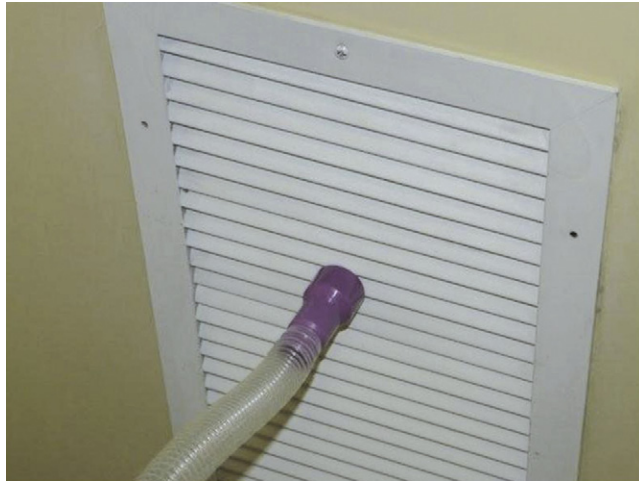
FIGURE 5-14 ■ Exhaust grille adapter for passive disposal of waste anesthetic gases via the operating room ventilation system.
