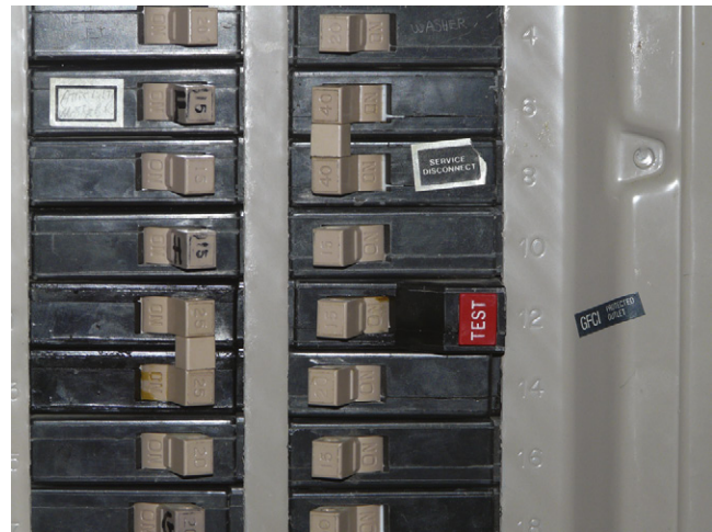
FIGURE 31-29 ■ Special ground fault circuit interrupter circuit breaker. Note the distinguishing red test button.
