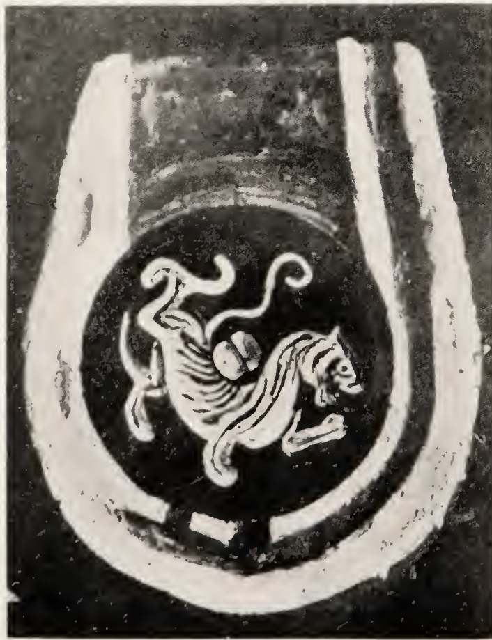
Sand-mould for casting the Han Mirror.
