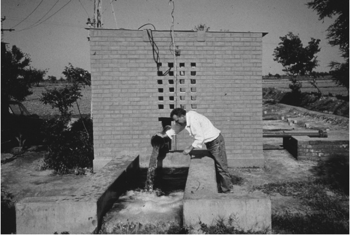
Figure 1.3 A dual purpose irrigation and drainage well in the Indus valley, Pakistan. In this ‘scavenger well’ the outlet pipe in the foreground of the picture is discharging fresh groundwater from the upper part of the well, whereas the pipe to the right is discharging saline water from the lower section of the well, thus preventing the saline water from moving upwards and contaminating the good quality water. The good quality water is used for irrigation whilst the saline water is diverted to the drainage system. Photo by Bruce Misstear
