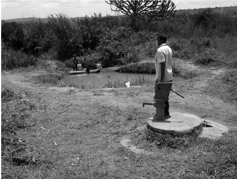
Figure B3.9(i) A broken hand pump over a well in Uganda, with people reverting to an unprotected water source in the background. Photo by Bruce Misstear
