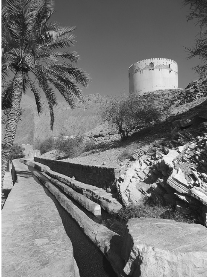
Figure 1.1 Open section of falaj (qanat) running through a town in northern Oman. Here, the channel is divided into three, with two of the channels then rejoining (at the bottom of the picture), in order to produce a two-thirds: one third split in the flow downstream. This Falaj al Khatmeen is included on the UNESCO list of World Heritage Sites. Photo by Bruce Misstear
