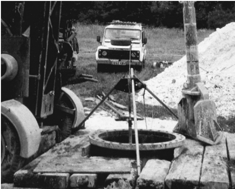
Figure 6.20 Photograph of the geophysical logging of a Chalk well in Southern England. Note the chisel of the cable-tool percussion drilling rig. Note also the logging cable emerging from the front of the vehicle and running over a pulley into the well. Photo by David Banks
