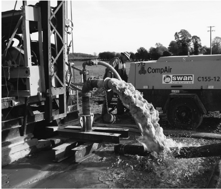
Figure 5.27 Well development using air-lift pumping, Ireland. Photo by Bruce Misstear
