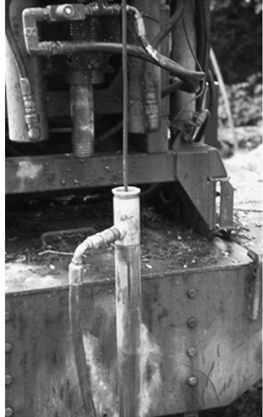
Figure 5.10 Retrieving core using the wireline system, western Ireland. Photo by Bruce Misstear
