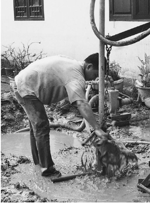
Figure 5.22 A well being drilled by jetting, Indonesia. Photo by David Banks
