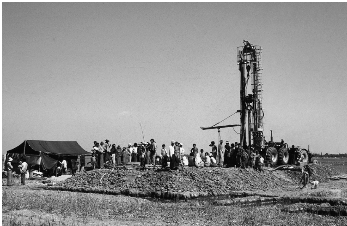
Figure 5.14 Tractor-mounted rotary rig raised above the ground surface in order to provide the necessary hydrostatic pressure for reverse circulation drilling. The target aquifer in this area of central Myanmar had a potentiometric surface only about 1–2 m below ground level. Photo by Bruce Misstear
