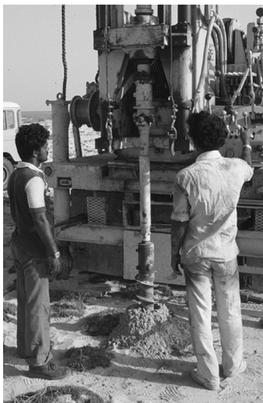
Figure 5.20 Hollow-stem auger drilling, Saudi Arabia. Photo by Bruce Misstear
