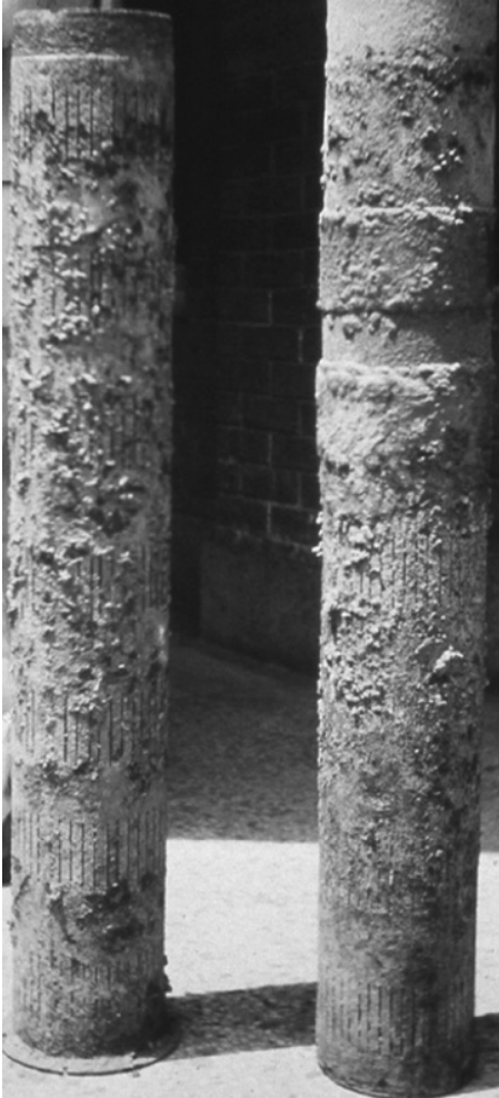
Figure 9.1 Encrusted well screens, Pakistan. The characteristic iron oxide 'tubercles' are visible on the surface of these steel screens. Photo reproduced by permission of Mott MacDonald Ltd
