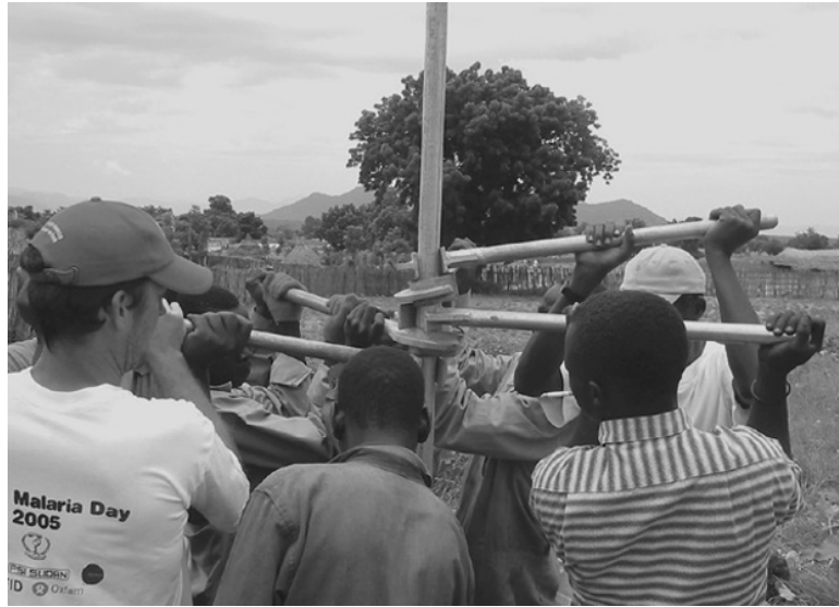
Figure 3.29 Removal of pump rods during hand-pump maintenance, Southern Blue Nile province, Sudan. Photo reproduced by permission of Laurence Gill
