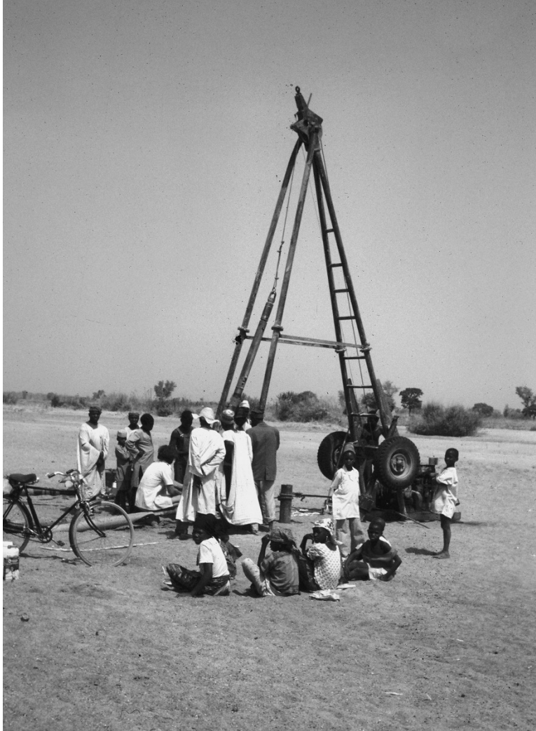
Figure 5.5 Light-percussion rig, northern Nigeria. Photo by Bruce Mistear
