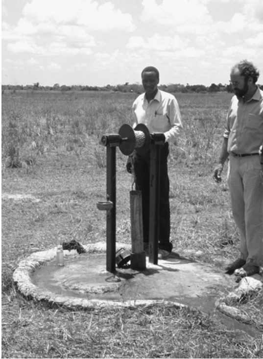
Figure 3.26 Bailer tube used in a rural Kenyan drilled well. Photo by David Banks
