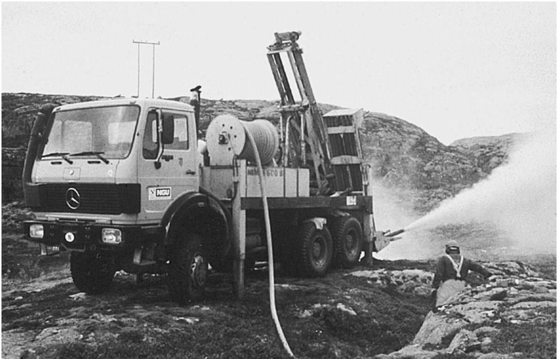
Figure 5.16 An inclined borehole being drilled by the down-hole-hammer method, Norway. Photo by David Banks
