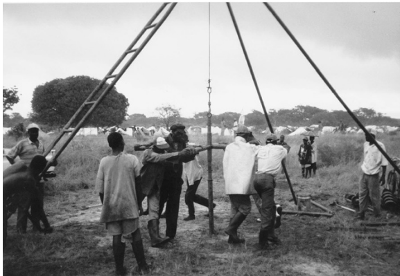
Figure B5.5(i) Drilling at (left) the Chiaquelane camp for displaced persons, and (right) a village near Chokwe, Mozambique, after the devastating floods in 2000, using the Vonder rig. The left hand photo shows drilling by manual rotation of the drill-string using a crossbar. The right hand photo shows the flight-auger bit and the temporary casing, and the rig’s winch. Photos by David Banks
