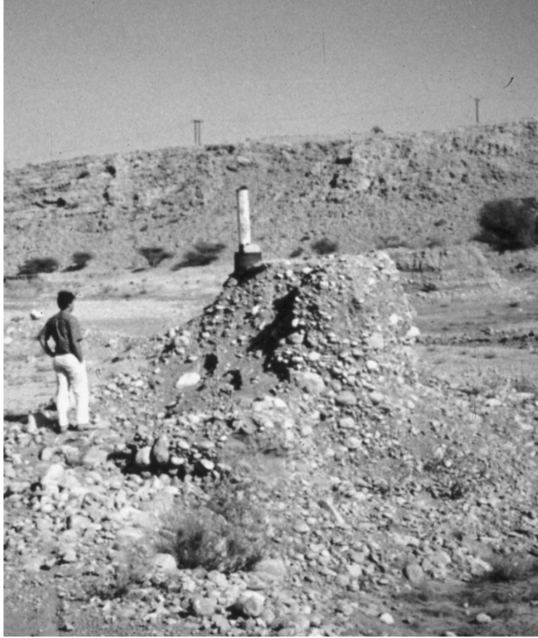
Figure 2.8 The remains of a well located in a wadi in northern Oman. The original wadi surface is preserved as a remnant mound around the top of the well casing. From the height of the hydrogeologist standing nearby, we can see that the wadi floor has been lowered by about 2 m due to erosion from the occasional, but violent, floods that occurred in the 20 year period between well construction and when this photo was taken. Photo by Bruce Mistear
