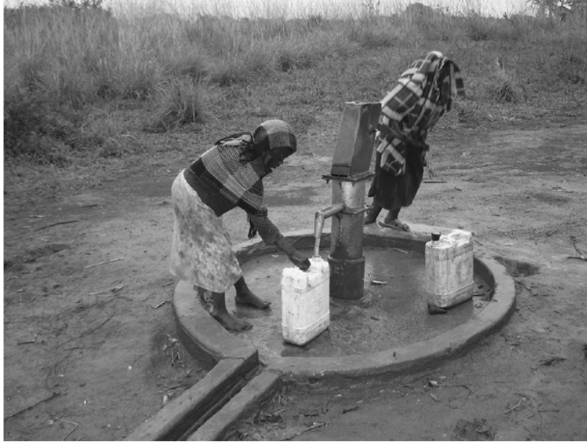
Figure 3.10 Concrete apron and drainage channel around a hand-dug well, Uganda. Photo by Bruce Misstear
