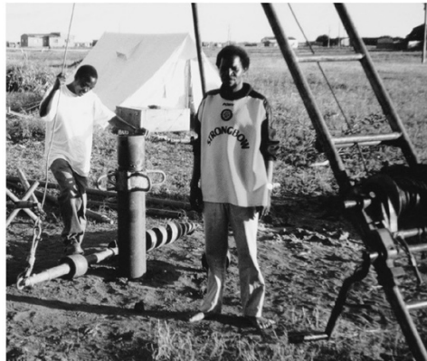
Figure B5.5(i) Drilling at (left) the Chiaquelane camp for displaced persons, and (right) a village near Chokwe, Mozambique, after the devastating floods in 2000, using the Vonder rig. The left hand photo shows drilling by manual rotation of the drill-string using a crossbar. The right hand photo shows the flight-auger bit and the temporary casing, and the rig’s winch. Photos by David Banks
