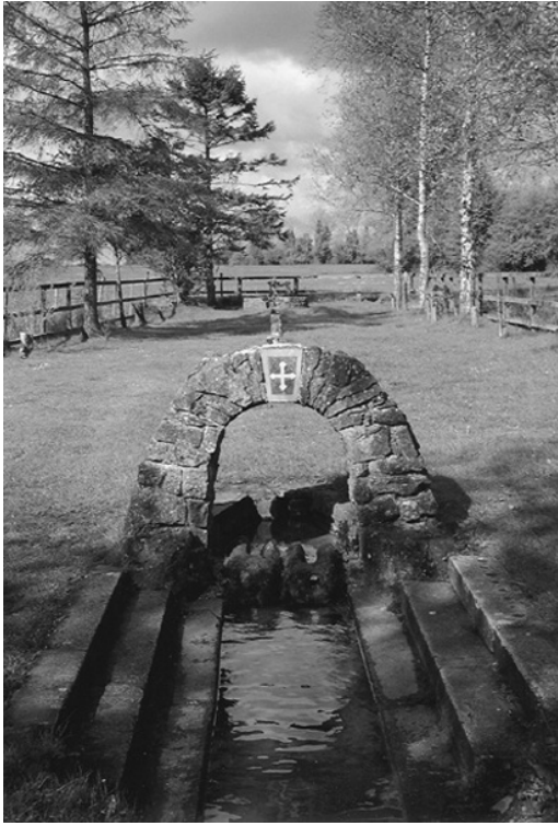
Figure B3.7(iv) St Brigid's well, County Kildare, Ireland. The well is located at the rear of the fenced area, behind the arch adorned with the white cross. The well is constructed around a small spring in a gravel aquifer and its discharge is channelled through two hollowed stones under the arch. The tree with the votive offerings shown in Figure B3.7(iii) is the second large tree from the left at the top of the picture. Photo by Bruce Misstear
