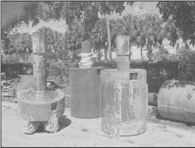
Figure 3-17 Three stabilizers and a 42-in. drill bit (left)
