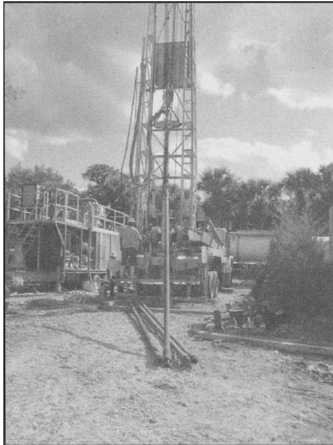
Figure 3-18 Picking up drill pipe
