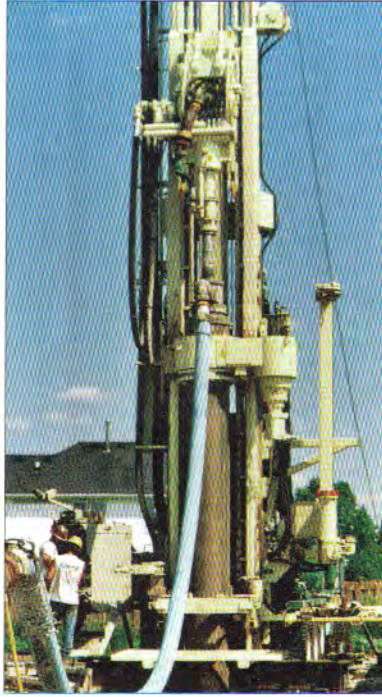
Figure 7.15. Casing rotator rig (Schramm, Inc.).
