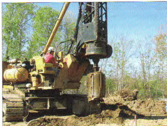
Figure 7.22. Bucket auger drilling rig (Powers et al. 2007).
