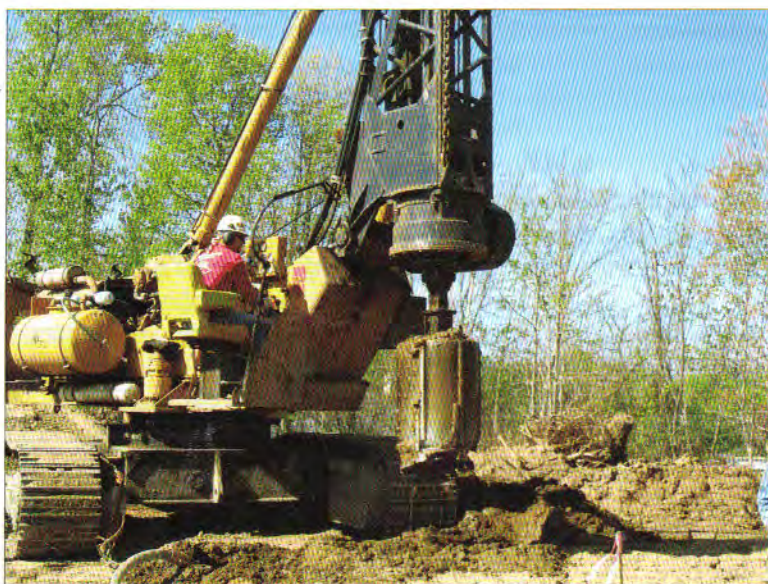
Figure 15.16. Bucket-auger drilling using a large truck-mounted foundation drill (Moretrench).
