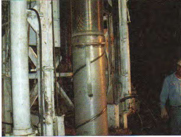
Figure 10.19. Centralizer on a screen (Clear Creek Associates).
