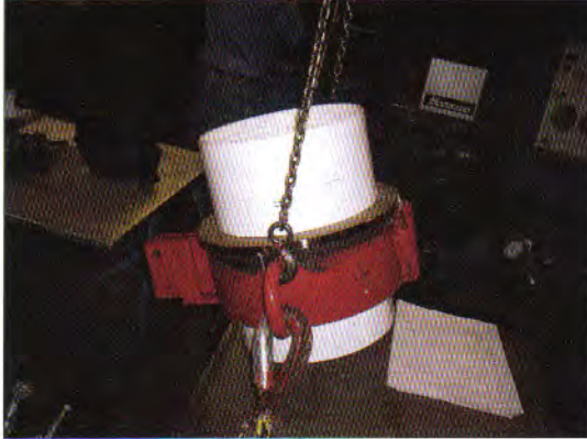
Figure 10.25. Elevator holding PVC pipe.
