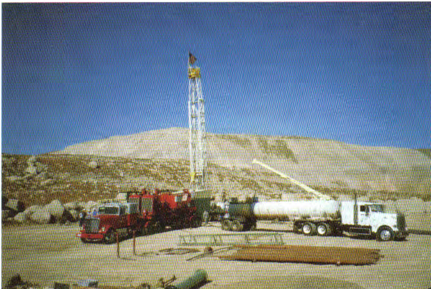
Figure 11.26. Acid is pumped into well to open fractures in a limestone aquifer.
