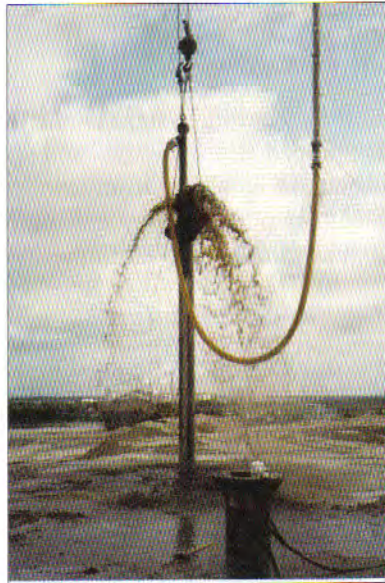
Figure 15.15. A jetted well installation (Moretrench).
