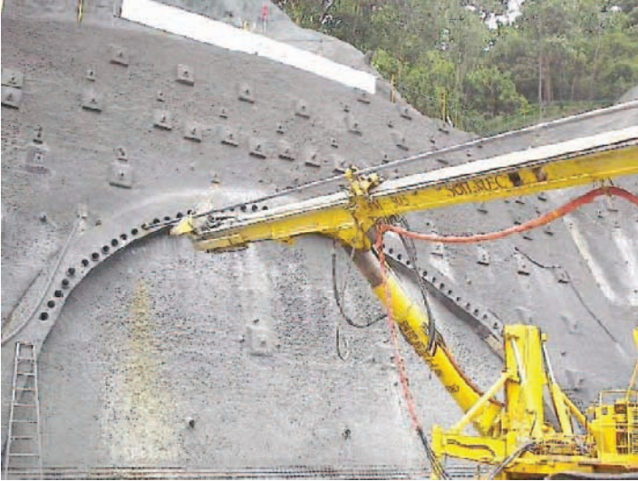
Figure 11.2 Installation of Pipes Above Portal
