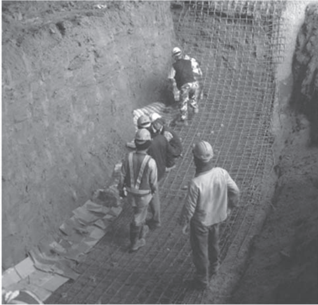
Figure 13.6 Installing Rebar for Final Invert
