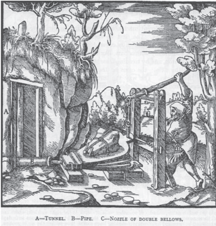
Figure 16.1 Early Mechanical Ventilation Using Bellows (Agricola, 1556)
