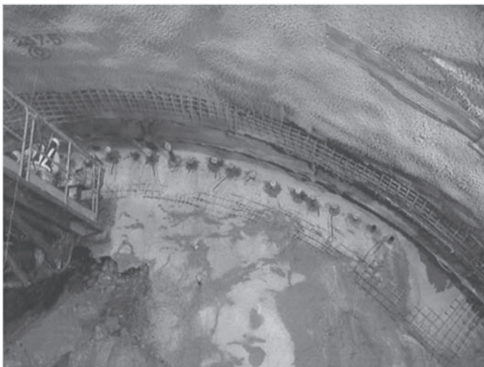
Figure 13.11 Grouting Pipe Roof
