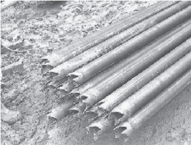
Figure 11.3 Pipes Cut To Facilitate Installation
