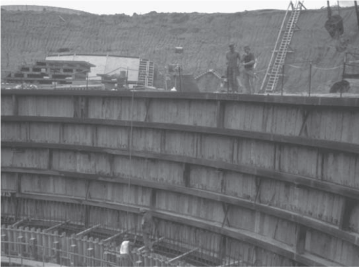
Figure 11.12 Ribs and Lagging for Shaft Support (Courtesy of Photographer: David Sailors)
