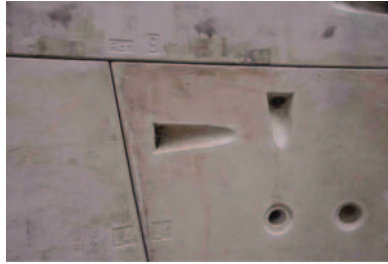
Figure 17.8 Bolt holes in segment
