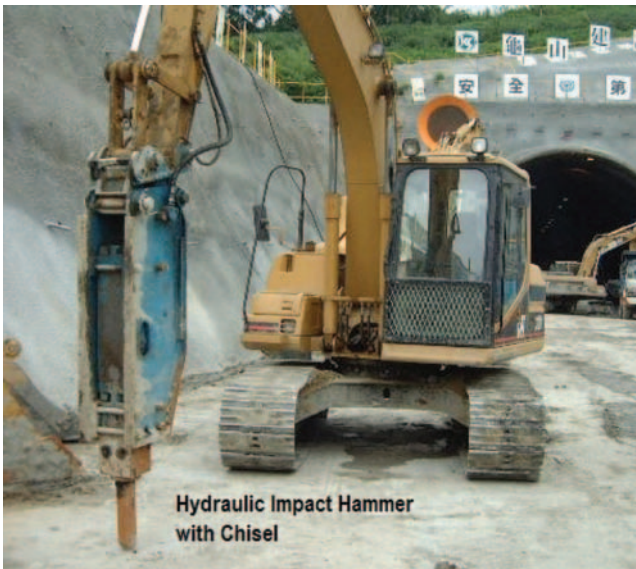
Figure 5.33 Impact Hammer Mounted on Excavator Boom
