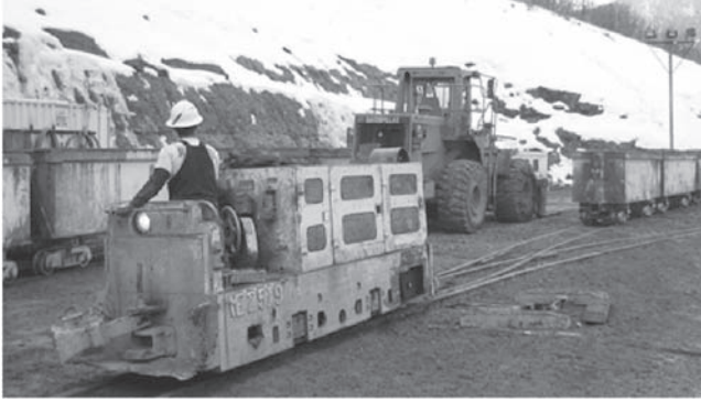
Figure 9.7 Locomotive Positioning to Couple to Muck Cars
