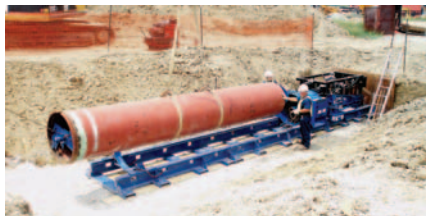
Figure 15.2 Auger Boring Machine with Casing and Cutterhead (Courtesy of American Auger)
