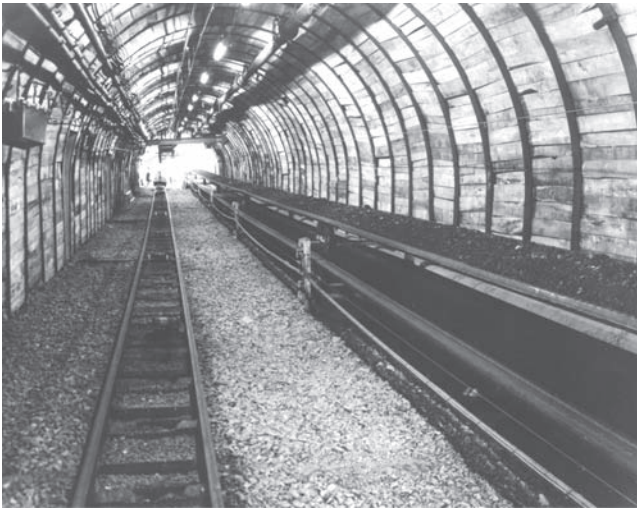
Figure 8.12 Ribs Using Wood Lagging (Note conveyor on lower right and rail at lower left.) (The National Archives, Her Majesty’s Stationery Office, United Kingdom)
