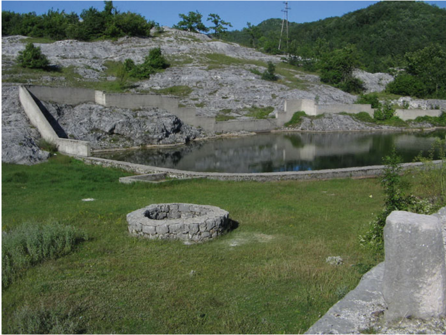
Fig. 5 A cistern-reservoir of rainwater and a well in the high karstic mountains of (Vilusi, Montenegro; published by Stevanović [3], Springer’s copyrights)
