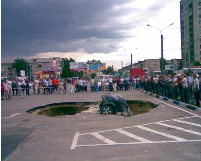
Fig. 4.2 Development of a karst-suffosion sinkhole induced by a heating main leakage in Dzerzhinsk (2009)
