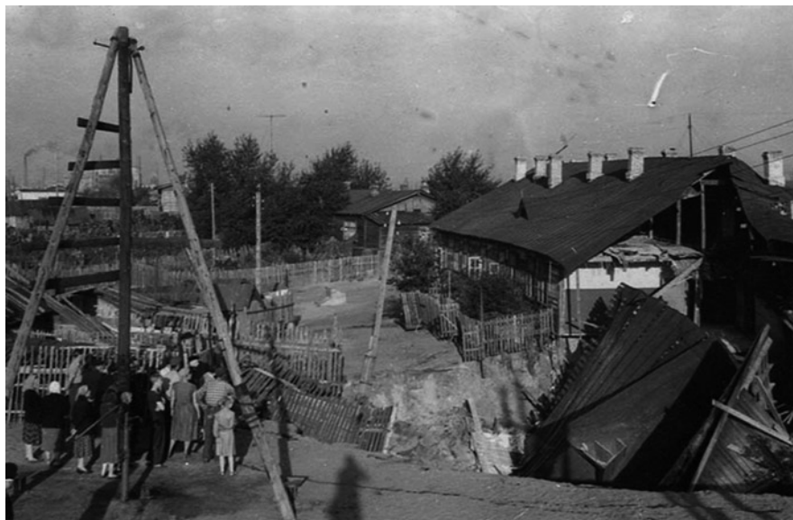
Fig. 4.3 Collapse of a residential building in Nizhny Novgorod region (1959)
