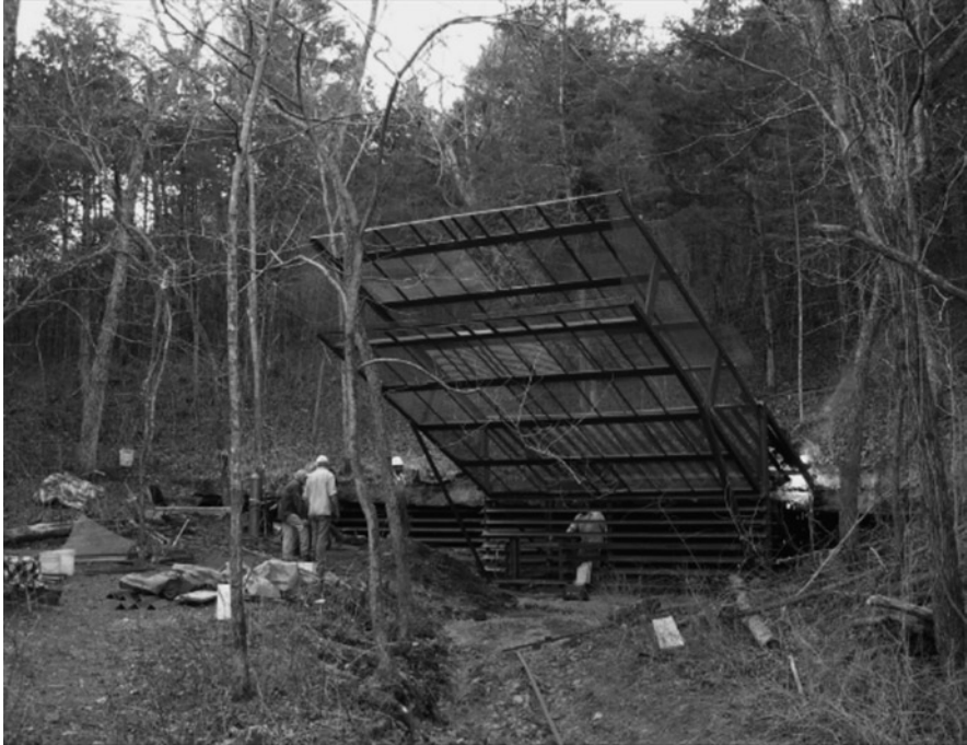
Fig. 6.2 Construction of the Tumbling Creek Cave chute gate, March 2004. The open chute allows pregnant gray bats to use the entrance freely, but excludes human intruders. Bats have increased in numbers since the gate was built (From Elliott and Aley 2006)
