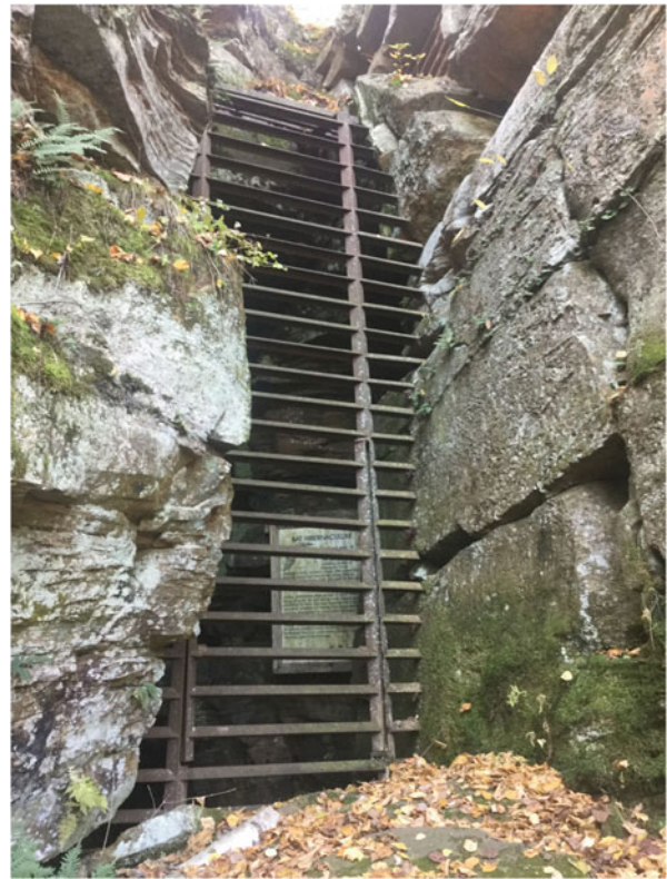
Fig. 3.50 Robinson’s Ice Cave bat protective gate with signage visible within. 2018 photo by Greg Brick
