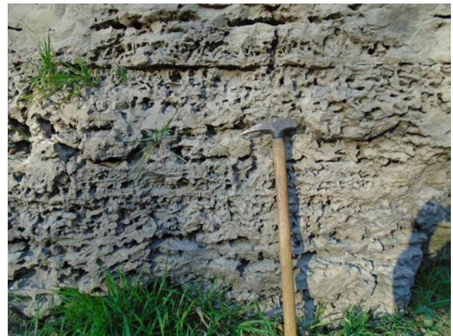
Fig. 7.13 Weathered east-west vertical extension fracture face illustrating the typical character of the Thalassinoides lithofacies. The raised areas are the dolomite burrow fills. The cavities are where calcite was dissolved during mineralization. The entire rock is dolostone. The exposure is of the upper portion of Prosser Fm. located at the mouth of Catfish Creek immediately below the Julien Dubuque Monument (42.468°N, 90.645°W). Rock hammer is 0.8 m long
