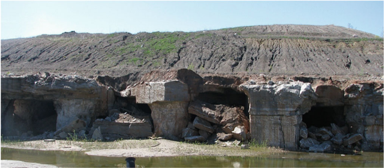
Fig. 4.28 Collapsed and partially collapsed mine drifts in the Gypsum Creek gypsum encountered during surface mining in the U.S. Gypsum Old Mill Meadows Mine (2010)
