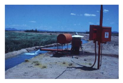
Fig. 5.6 Groundwater being pumped into a distribution canal
