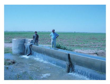
Fig. 5.5 In the distribution system the misdistribution of water usually exceeds seepage
