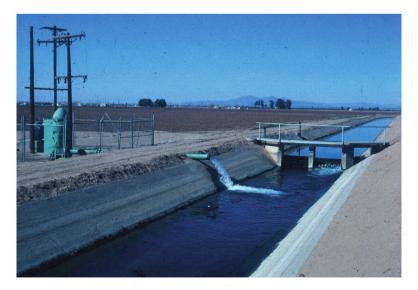
Fig. 5.10 Pumping groundwater into the (downstream) part of the conveyance systems improves the operational flexibility and control of the groundwater table
