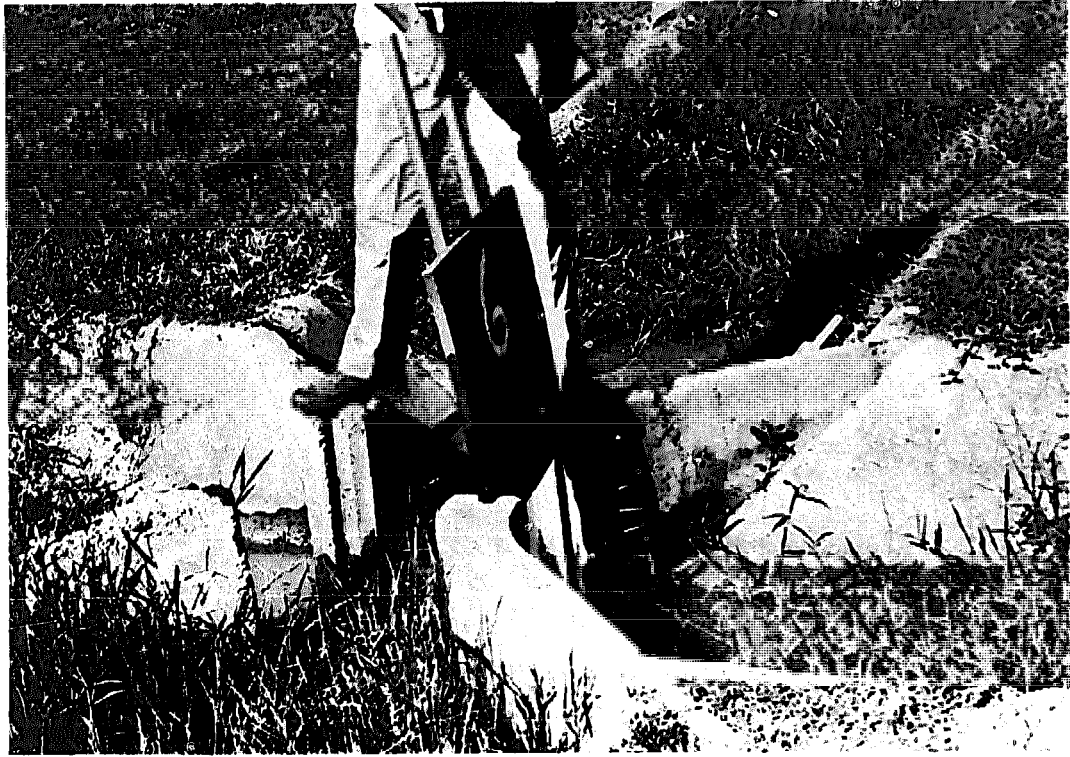
FIGURE 29. Concrete check gate placed in earthen ditch. Grooves permit using flashboards for checking flow of water, or directing the flow into different laterals.
