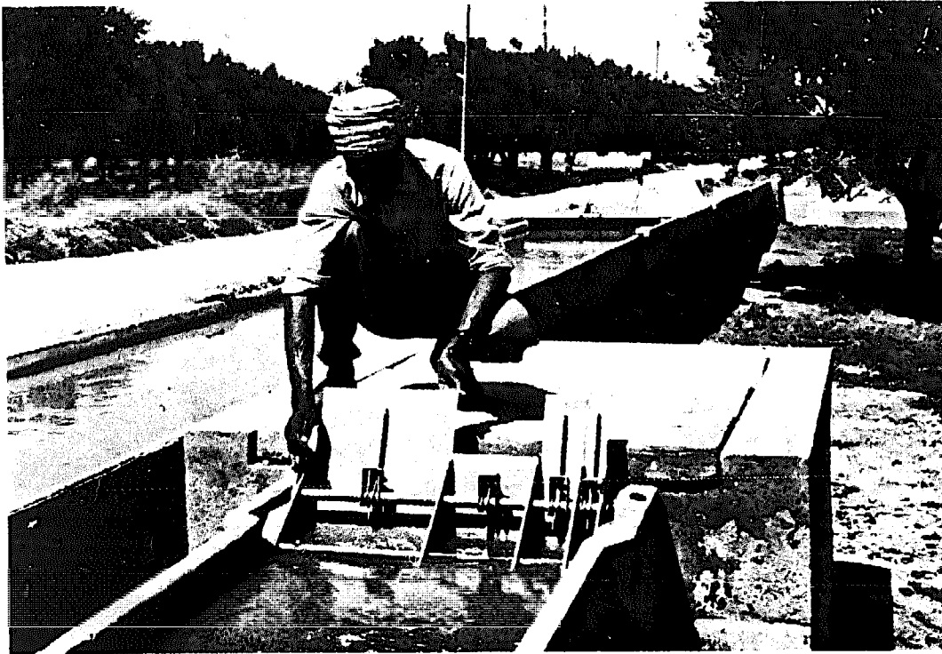
FIGURE 1. Distributor, with Neyrpic automatic gate downstream in the main canal to regulate water depth.
