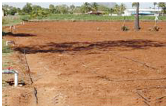
Installation of drip irrigation system
