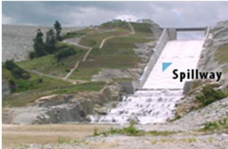
Fig. 13.2. Chute spillway.
