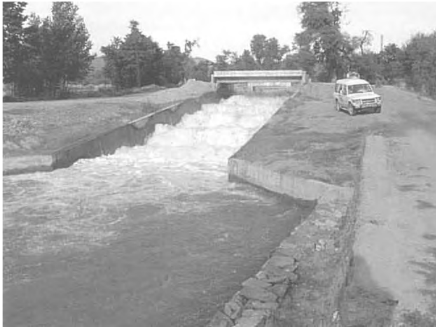
figure 7.12 Baffled chute drop
