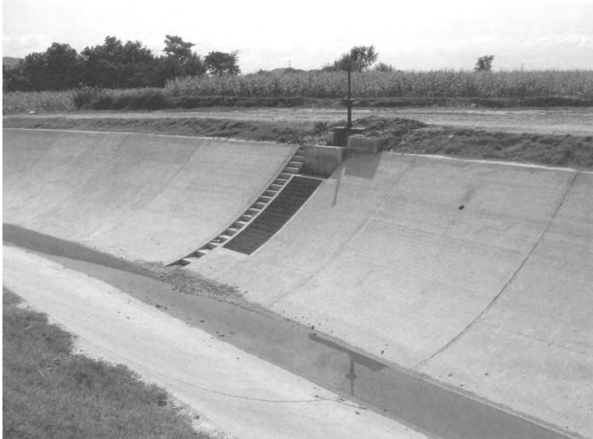
figure 8.14 Pipe intake from a level-top canal
