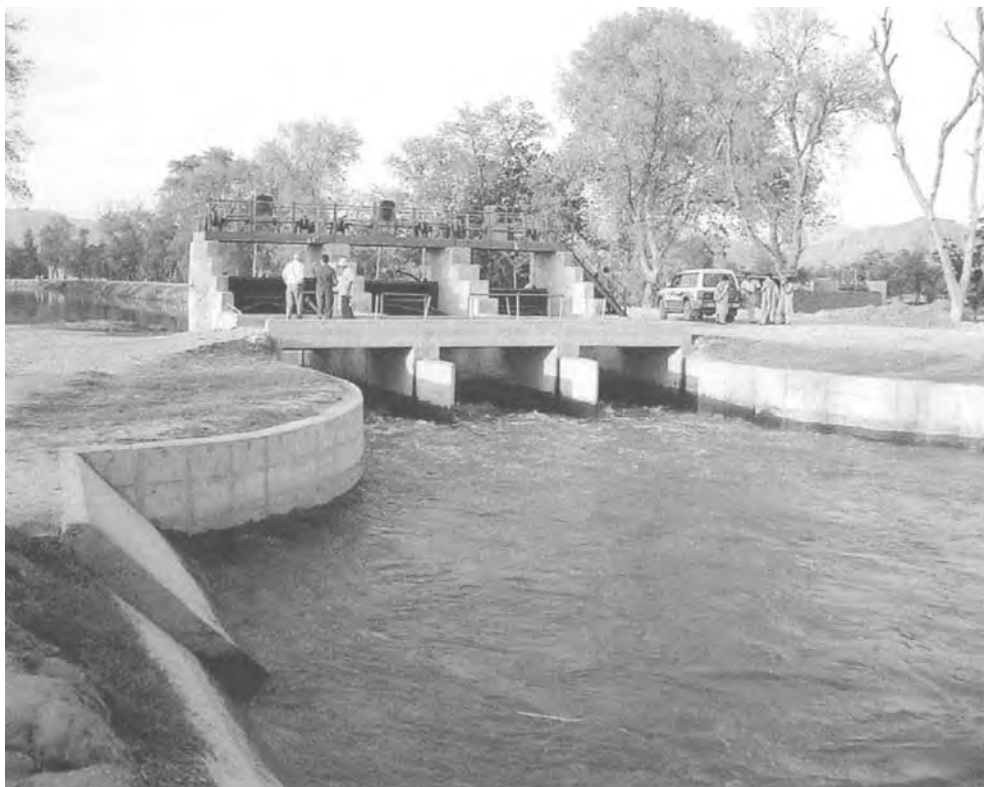
figure 3.6 Cross regulator on Machai Branch
