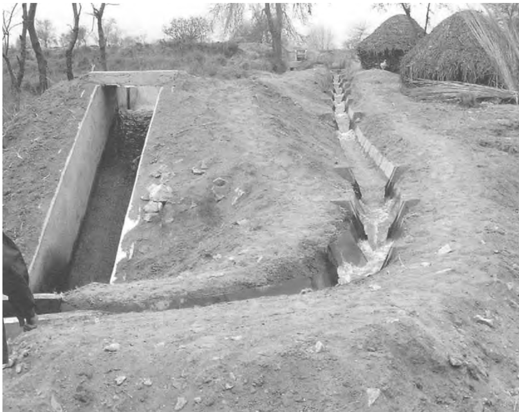
figure 7.15 Stepped Drop cascade in a parabolic watercourse, and a glaciis drop in its parent distributary.
