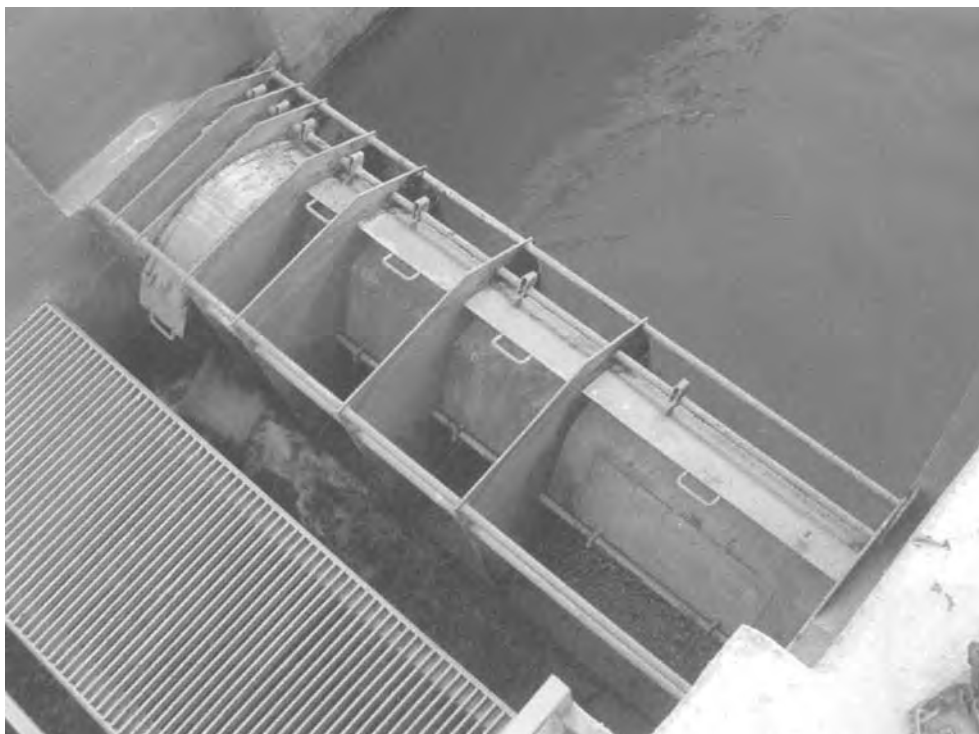
figure 4.15 Modular distributor
