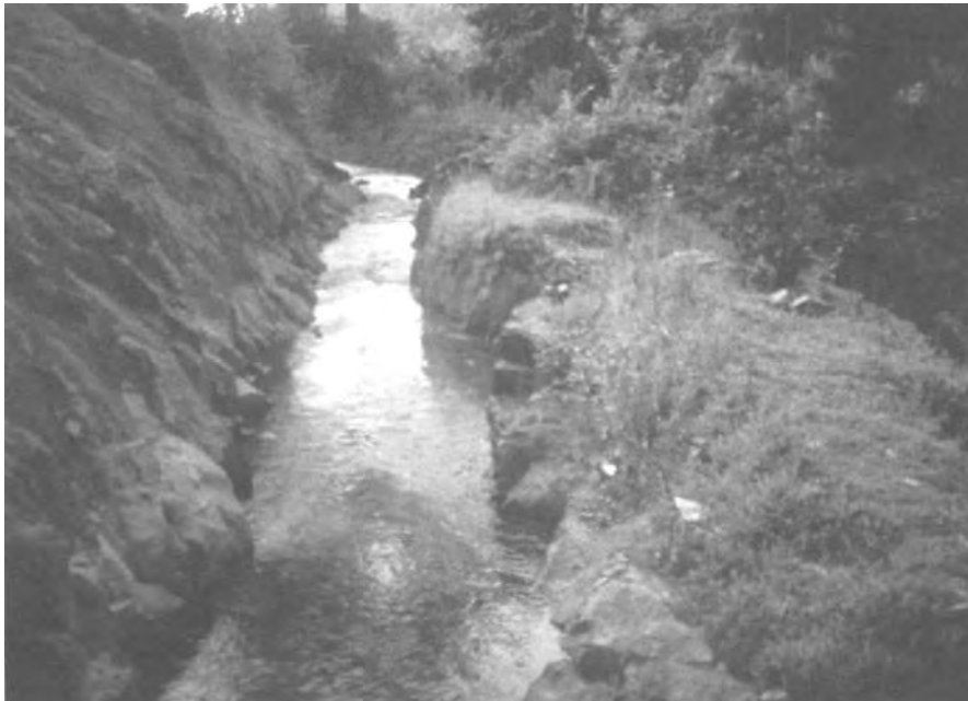
figure 11.3 Bogribail Canal through rock
