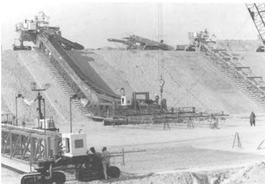
figure 9.7 Slip forming the Ghazi-Barotha power canal, Pakistan
