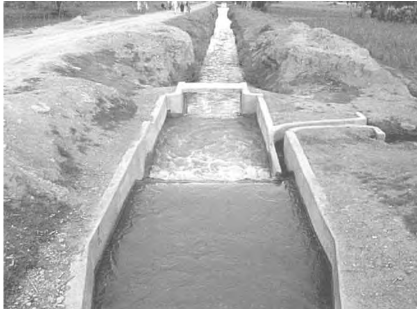
figure 4.14 A proportional divider abstracts a fixed proportion of the flow in the parent canal
