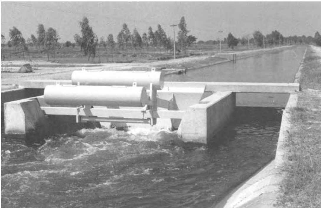
figure 4.2 Upstream control by a float-operated self-regulating gate, Thailand (courtesy Wolfgang Stenzel)
