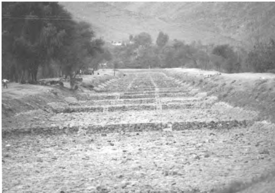
figure 10.2 A rough canal. The Pitched Channel of the Upper Swat System, Pakistan. This was intentionally designed as rough as possible in order to control the velocity over its 4 mile length. Slope of the channel is 1 in 100, with additional ramp falls shown at intervals of between 10 and 30 metres. Manning's n is estimated at 0.025.
