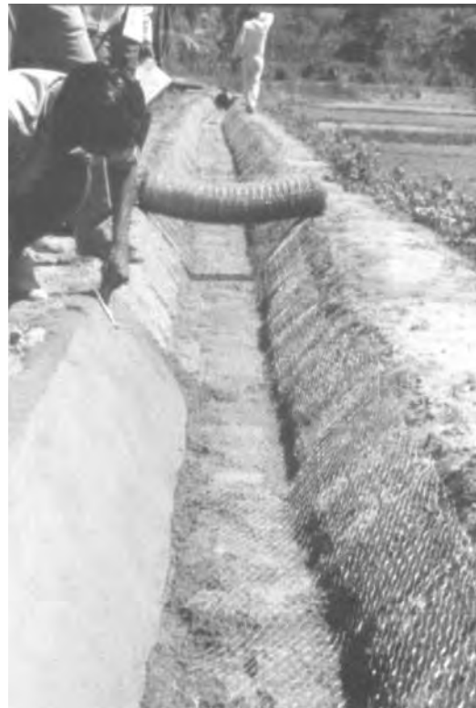
figure 9.9 Laying ferrocement
