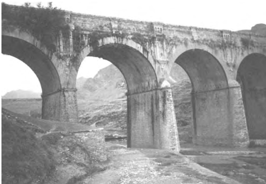
figure 1.1 Arch aqueduct on the Upper Swat Canal, Pakistan
