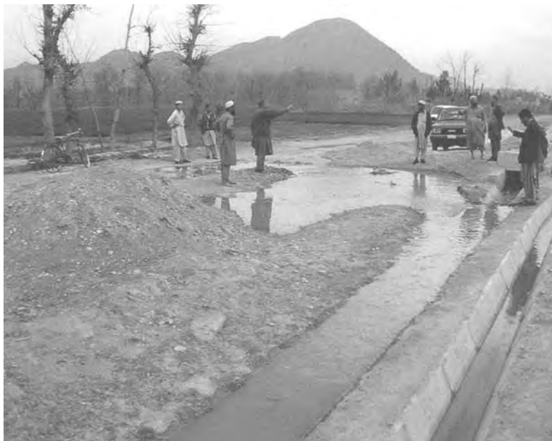
figure 5.5 Management losses from Zaida Minor flood the road in NWFP, Pakistan
