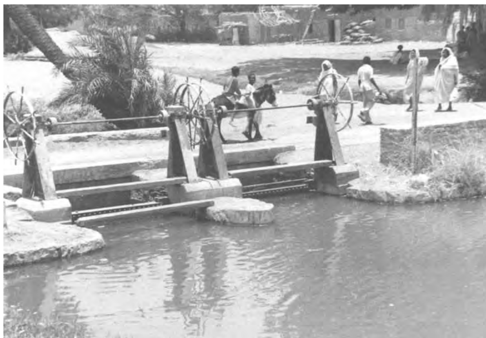
figure 1.3 A minor headsluice in the Gezira, Sudan. This scheme was built for commercial cotton production in the 1920s. It was well-engineered but has had its own severe problems, particularly of siltation
