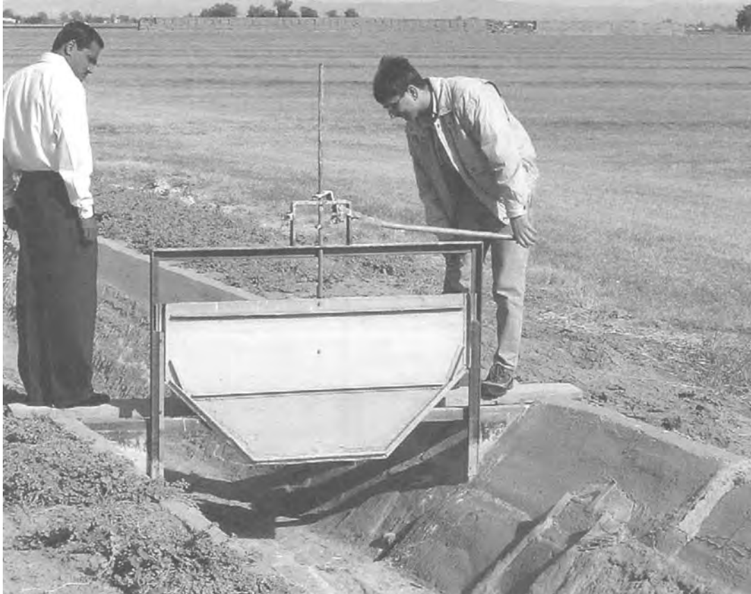
figure 4.7 A lever-operated check gate, Imperial Valley, California
