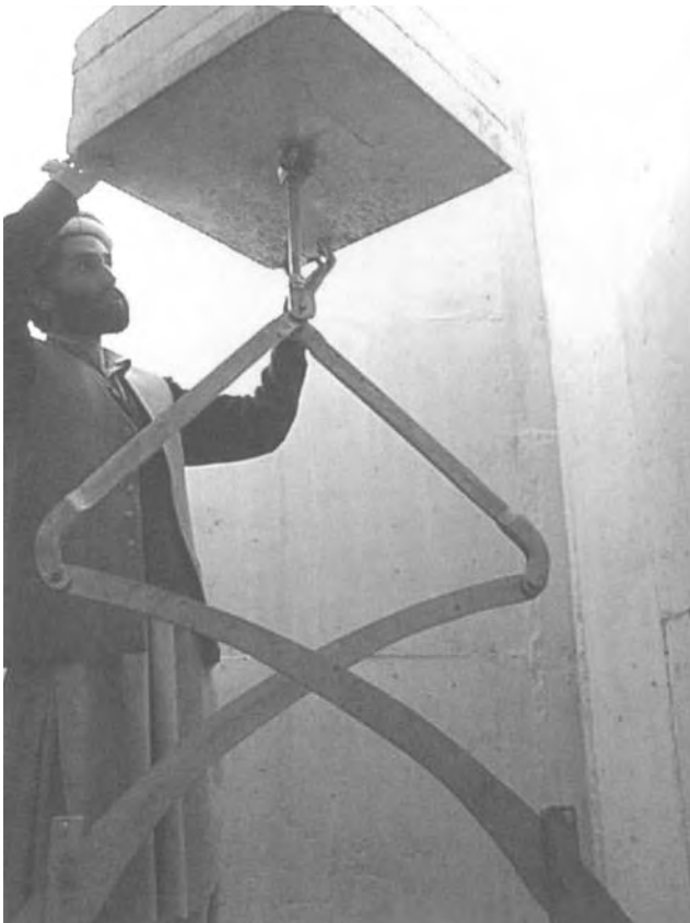
figure 8.10 Installing a Harris valve float
