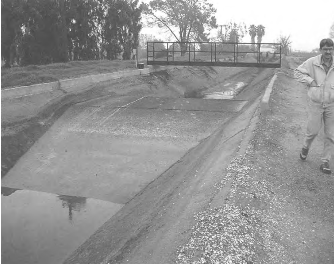
figure 7.24 A Replogle Weir at Patterson Irrigation Scheme, California
