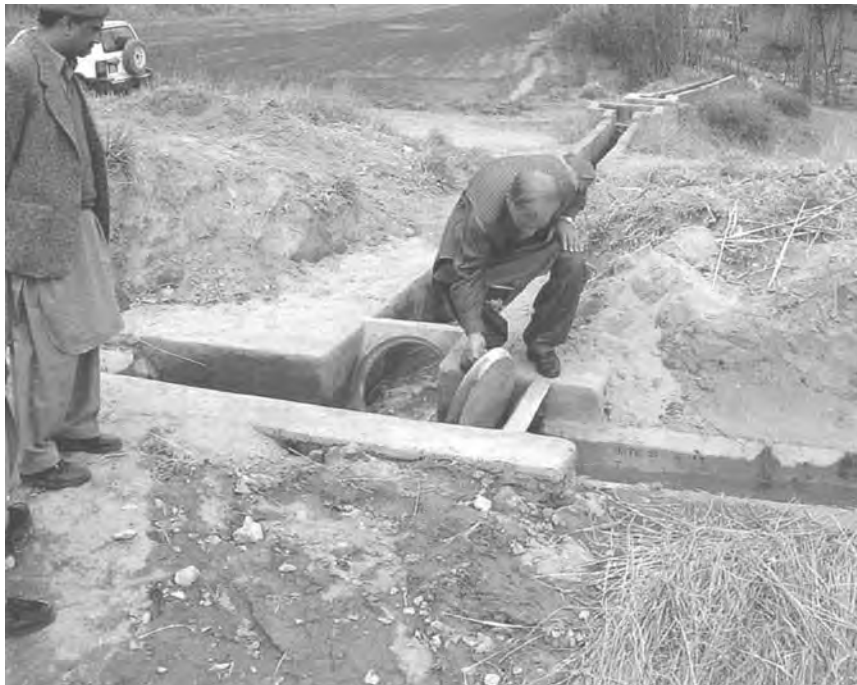
figure 6.4 Rectangular brick canal, Fakisian, with a pucca nucca outlet
