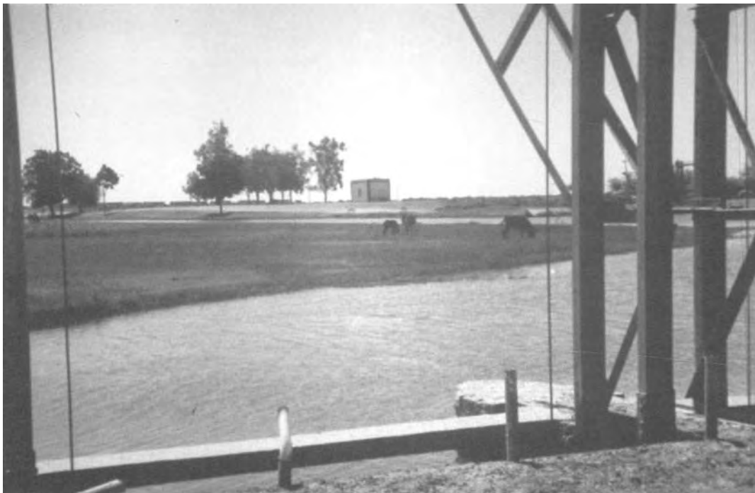
figure 7.29 Silt accumulation in a Gezira main canal, Managil extension, Sudan
