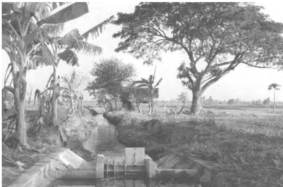
figure 7.5 Modular control gates (courtesy Wolfgang Stenzel)
