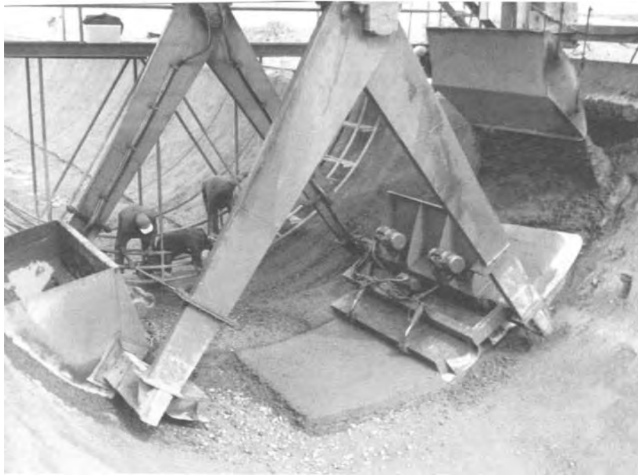
figure 6.6 Constructing a large circular canal, Spain (courtesy New Civil Engineer)
