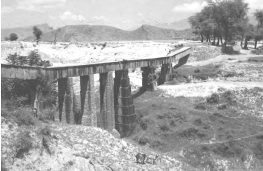
figure 7.20 Siphonic aqueduct, Shamozaï Distributary of Upper Swat Canal, Pakistan
