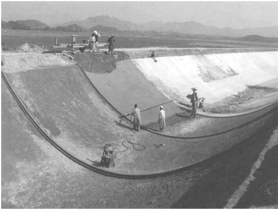
figure 9.6 Concrete placing on the Pehur High Level Canal
