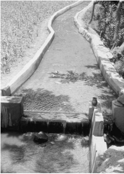
Fig. 4.33. Automatic proportional distribution on the main channel of a farmer-managed irrigation system in Nepal. Note the relative widths of the offtake on the right and the main channel.
