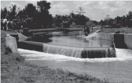
Fig. 4.32. Examples of orifice and weir combinations for flow control. (a) Gated orifice offtake with a duck-bill weir in the parent canal. Due to the extended length of the weir in the parent canal the head over the offtake orifice varies very little for relatively large variations in upstream discharge (Sri Lanka). (b) Diagonal weir in the parent canal with a set of Neyrpic offtake gates on the right-hand side (Morocco).
