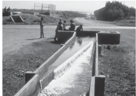
Fig. 4.32. Examples of orifice and weir combinations for flow control. (a) Gated orifice offtake with a duck-bill weir in the parent canal. Due to the extended length of the weir in the parent canal the head over the offtake orifice varies very little for relatively large variations in upstream discharge (Sri Lanka). (b) Diagonal weir in the parent canal with a set of Neyrpic offtake gates on the right-hand side (Morocco).
