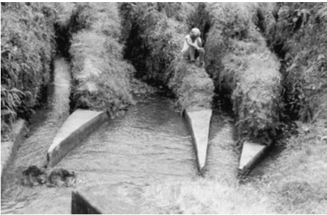
Fig. 4.10. Proportional flow control on farmer-managed irrigation systems on the slopes of Mount Kilimanjaro, northern Tanzania.
