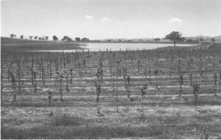
Figure 1.2 Large earthen dam storing water for irrigation. Detailed planning is essential to ensure successful construction and reliable inflows. (Courtesy Central Highlands Management.)
