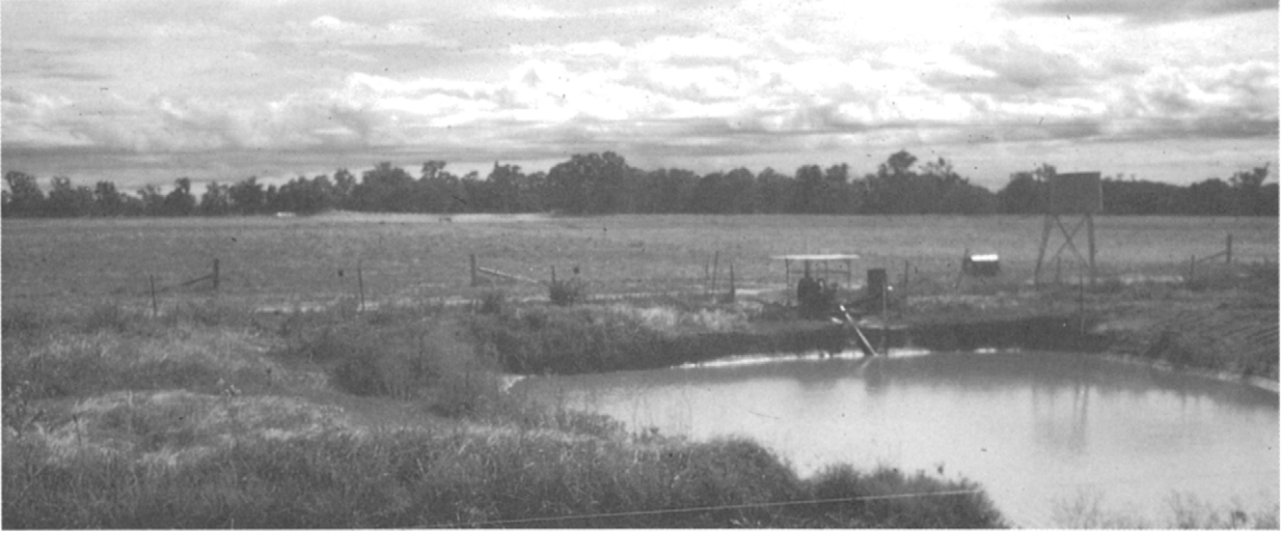
Figure 1.5 Tailwater from this border check irrigation system is delivered to a sump. From here, tailwater is pumped to a spray irrigation system, minimising environmental problems, and maximising use of water. (Water can also be supplied direct to the spray irrigation pump.)
