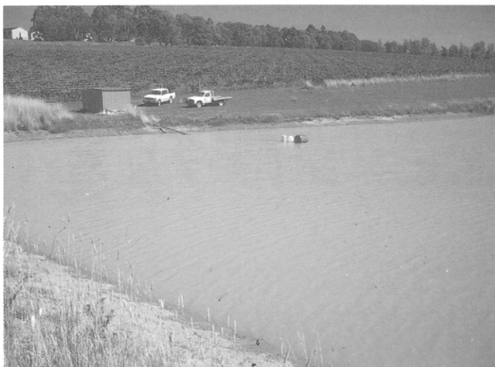
Figure 8.1 On this vineyard, the water supply and pump station are conveniently adjacent to the irrigated area, minimising costs of water reticulation. Water is delivered first to the top of the hill, then submains bring the water downhill to the laterals, to ensure even pressure to the laterals.
