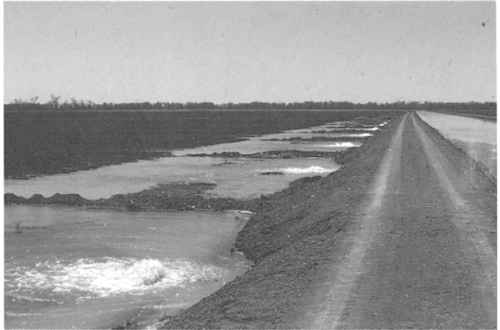
Figure 5.9 In this layout, a single large diameter outlet pipe services many furrows. The hinged gate on the pipe can be opened and closed from a vehicle, saving time.
