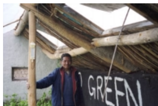
Picture 21 - View of white washed west wall and black painted north wall.
