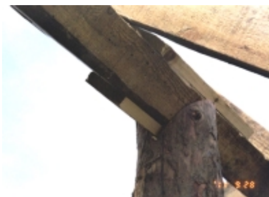
Pictures 30 & 31 - Beam fixation on the post in Ladakh (left) and Qinghai (right)
