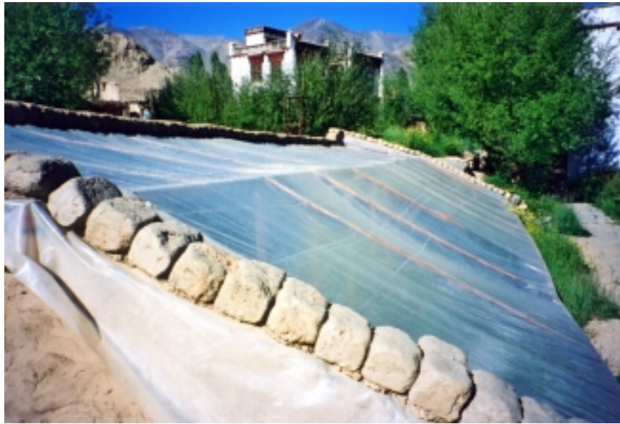
Picture 42 - Detail of polythene fixing by use of bricks laid on a mud coating.
