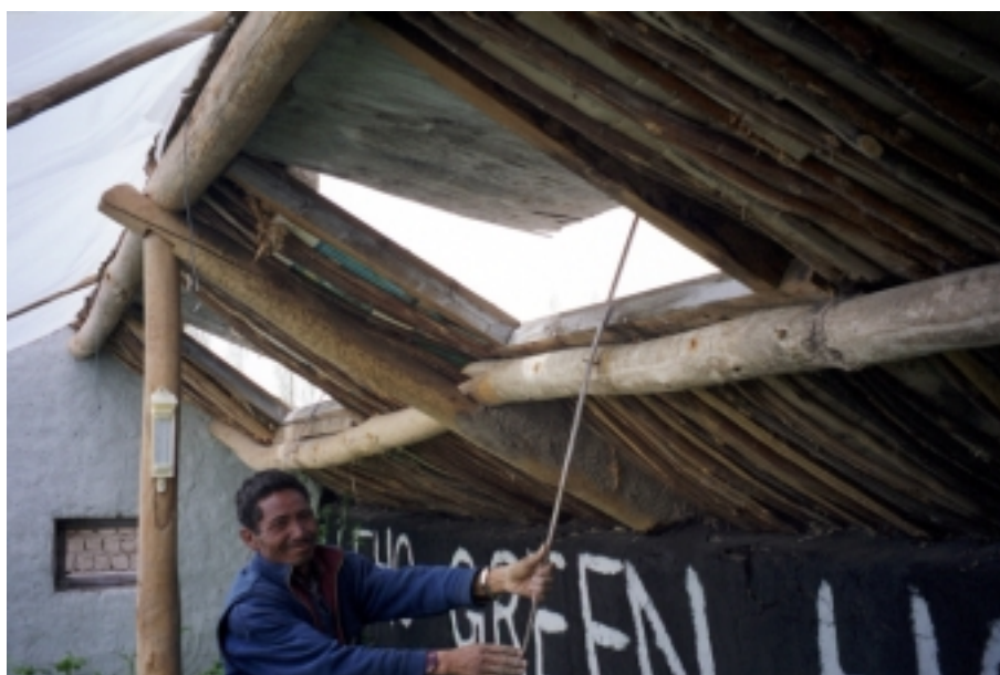
Picture 9 - Ventilator opening
