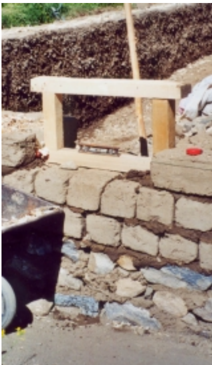
Picture 26 - Frame positioning on wall
