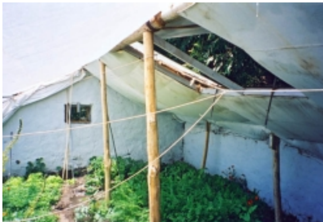
Picture 37 - White cloth under the roof
