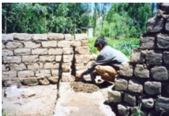
Picture 17 - Building of double wall with mud bricks in Ladakh
