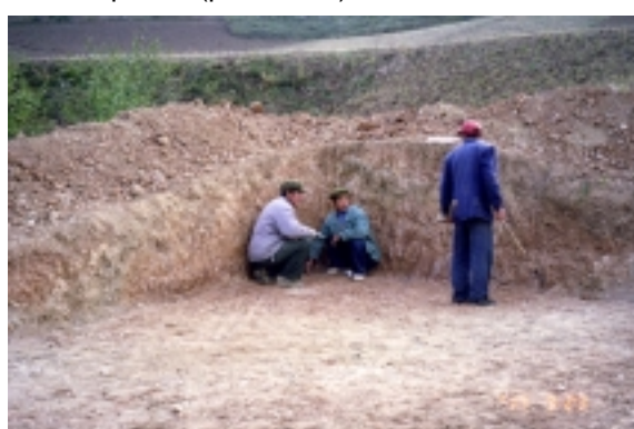
Picture 13 - Excavation of the slope
