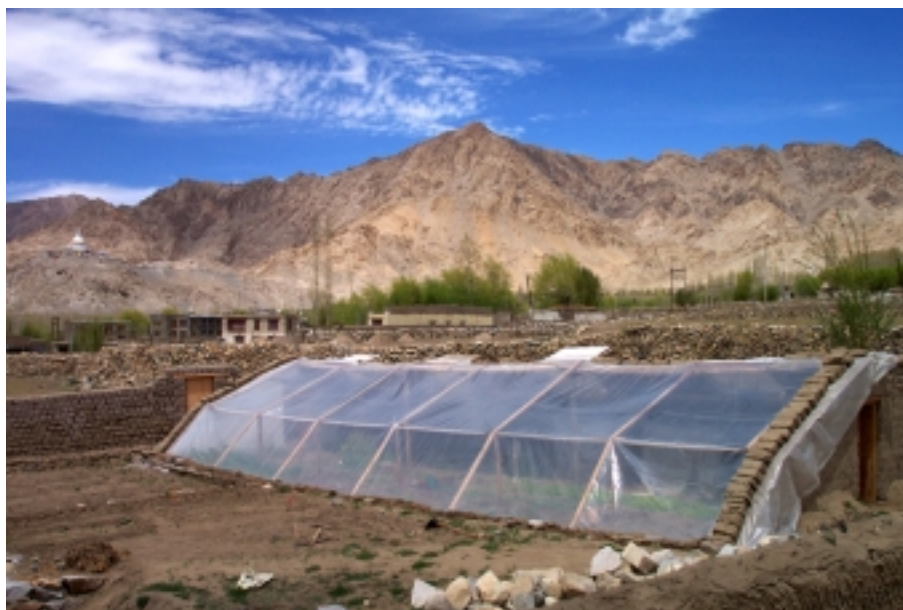
Picture 2 - Solar greenhouse built in Leh (Ladakh, India)
