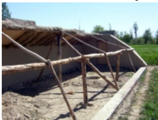
Picture 40 - Wooden structure to support polythene (Lowgar, Afghanistan)
