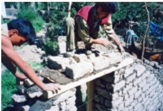
Picture 23 - Detail of the masonry procedure for building the doorway supporting wall
