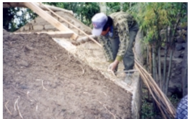
Picture 36 – Applying of cardboard, straw and Mud
