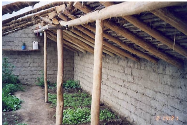
Picture 33 - One horizontal beam and several transversal joists in Spiti
