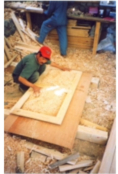
Picture 22 - Door construction
