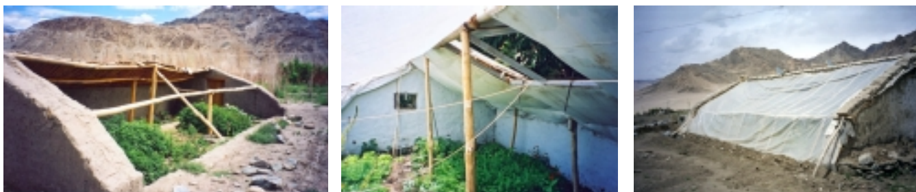
Pictures 5, 6, 7 - Greenhouse's structure
