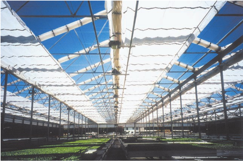
Photo 8.3. The retractable roof greenhouse can provide maximum ventilation.
