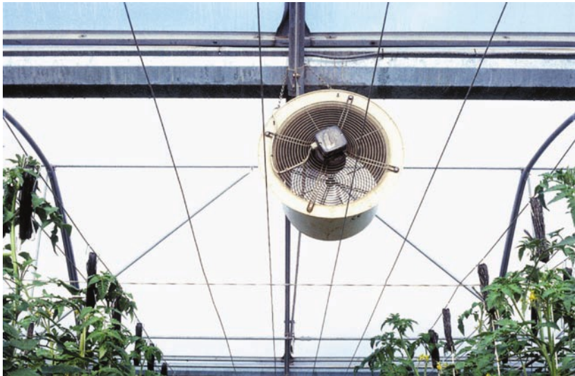
Photo 9.1. Destratification fans are increasingly used to mix the air in the greenhouse.
