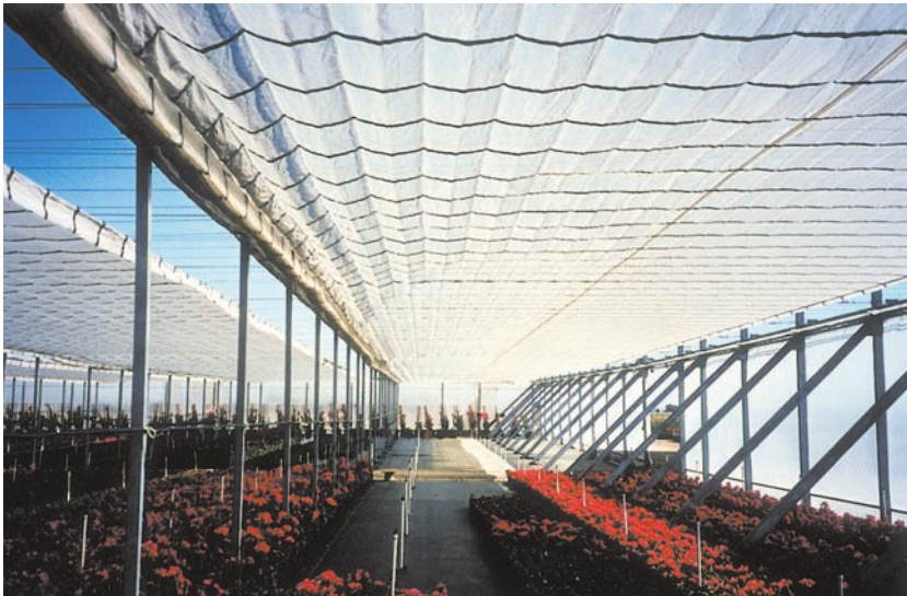
Photo 4.6. Retractable roof greenhouse (Cravo type) that permits the complete retraction of the plastic cover to maximize the solar radiation.
