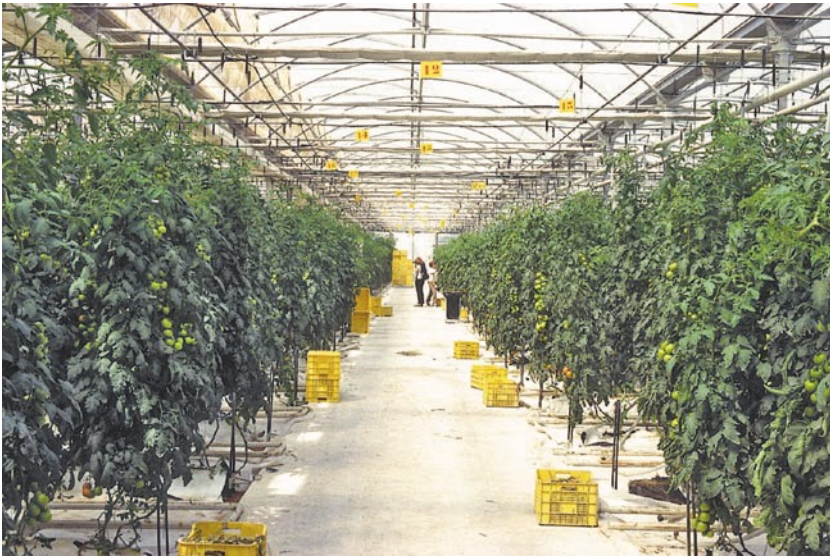
Photo 1.6. Plastic film multi-span greenhouse.
