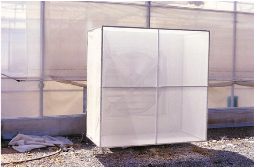
Photo 8.4. The injection ventilation fans must avoid the introduction of insects, by covering the air inlets, where external air is drawn inside, with proper screens.
