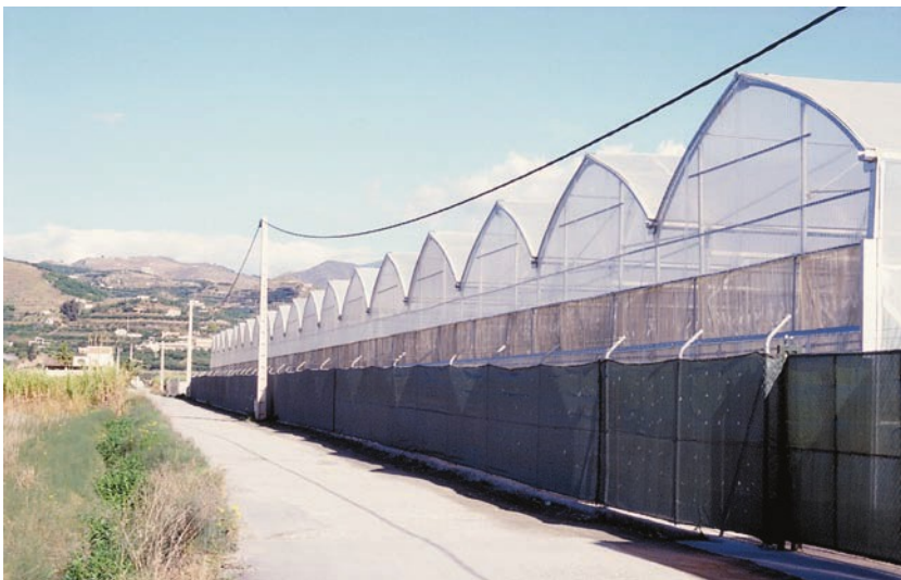
Photo 4.5. The steel structure is used in multi-span greenhouses.
