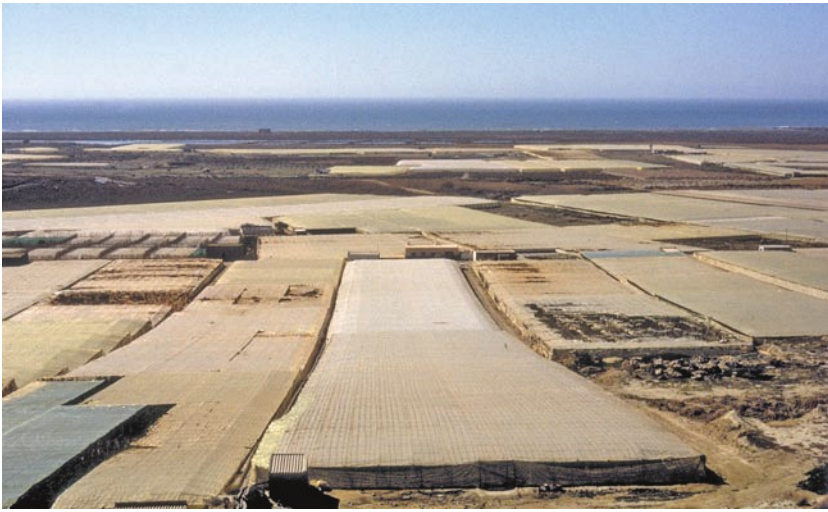
Photo 1.9. Plastic greenhouses in the Poniente area in Almeria; plastic greenhouses in Spain represent nearly 99% of the total greenhouse area.
