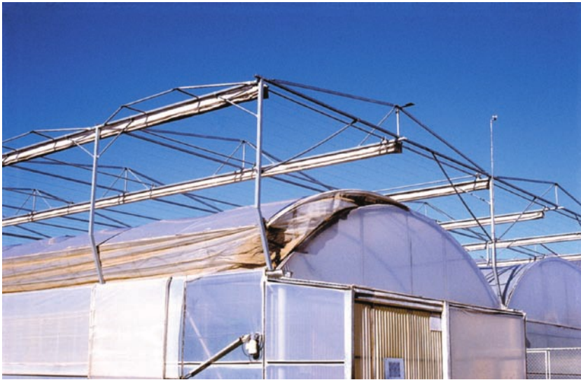
Photo 8.6. External shading device located over the greenhouse. The vents have anti-insect screens.
