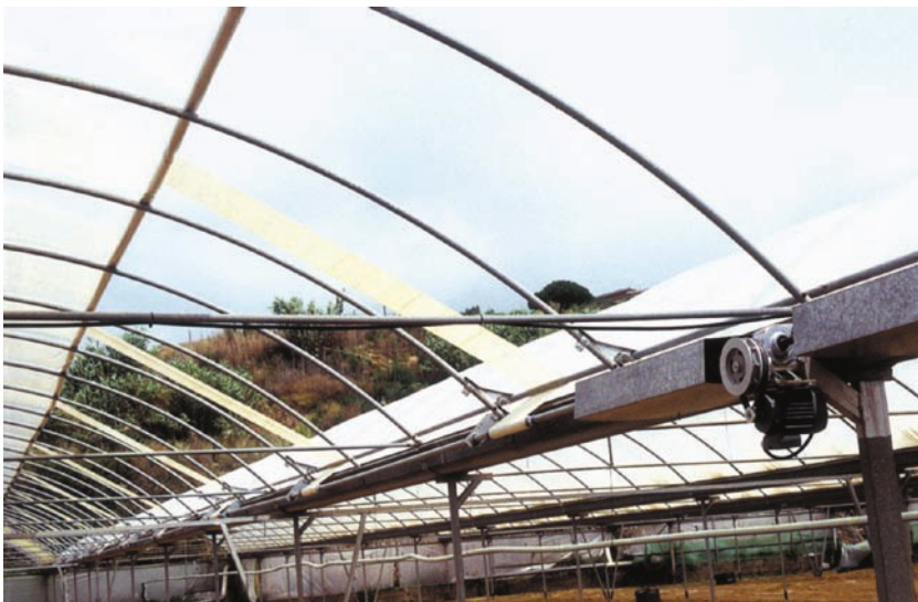
Photo 8.2. Rolling roof greenhouse (plastic film and screen) that allows the cover material to be selected depending on the climate conditions. (Source: J.I. Montero.)
