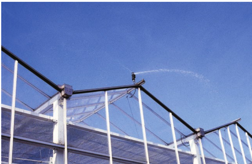
Photo 8.7. The 'irrigation' of the cover to cool the greenhouse has not been used in the Mediterranean.
