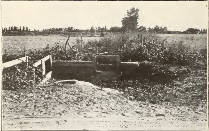
FIG. 1.—A BROAD, SHALLOW, WEED-COVERED IRRIGATION DITCH—THE USUAL CONDITION.
