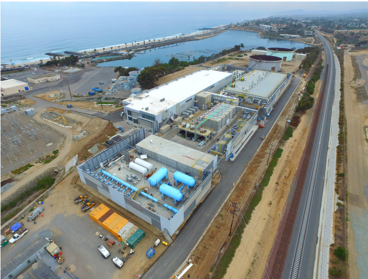
FIGURE 4.1 Aerial view of the 200-MLD Carlsbad SWRO desalination plant.
