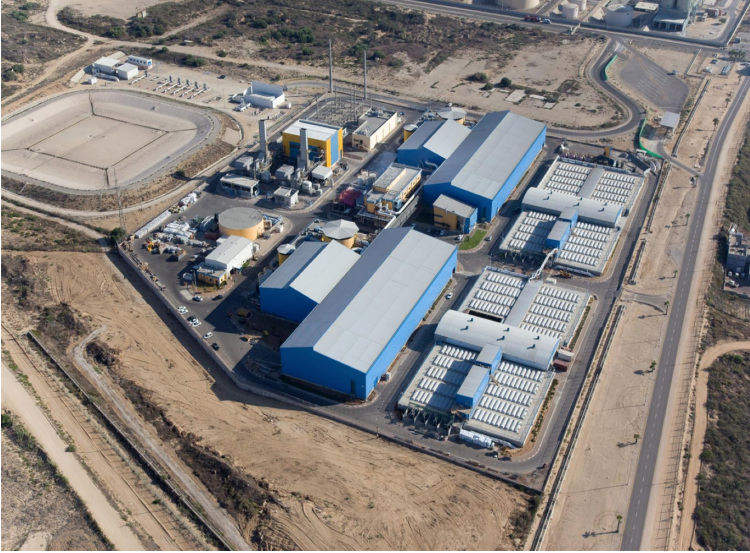
FIGURE 2.9 330-MLD Ashkelon SWRO desalination plant – aerial view.
