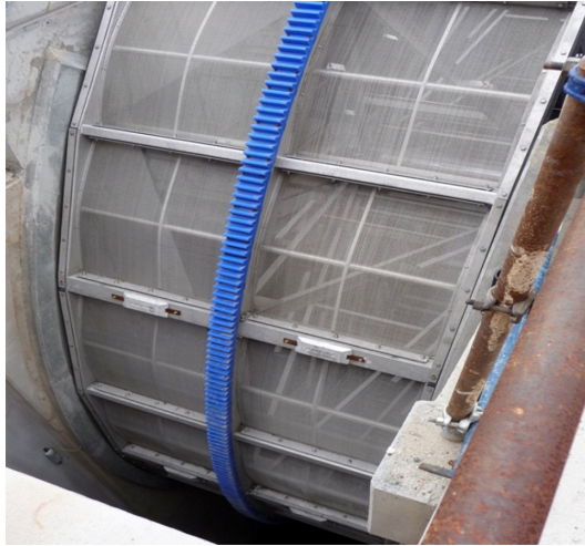
FIGURE 2.17 Fine intake screen.
