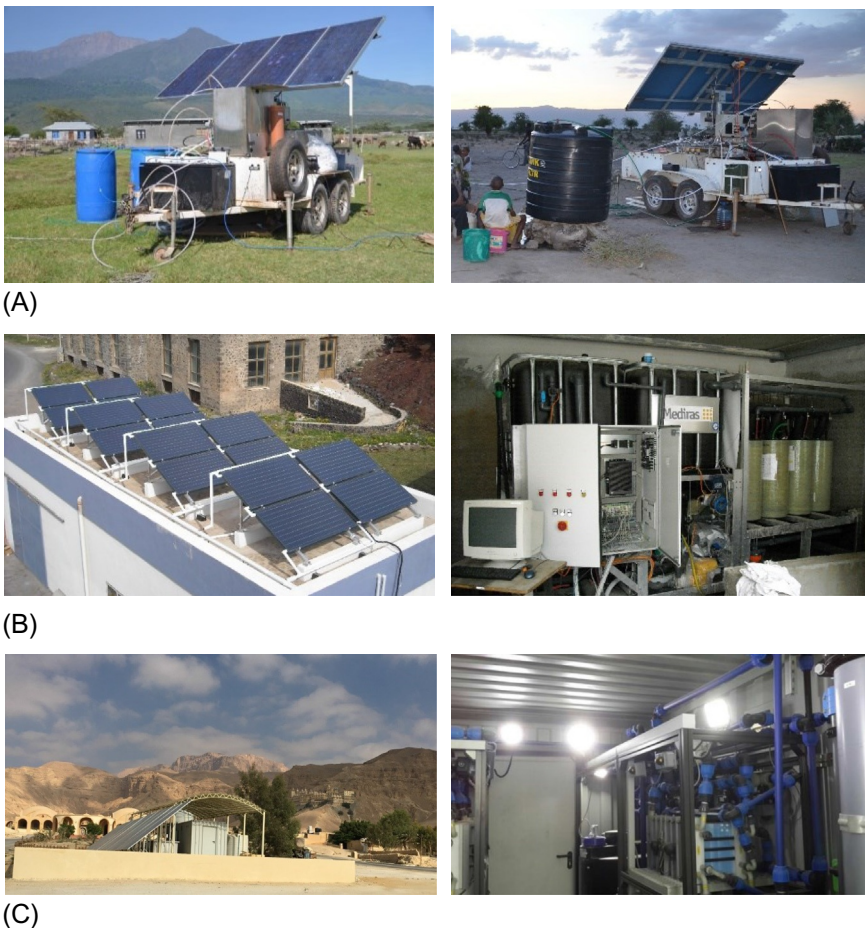
Fig. 11 Pictures of renewable energy-powered desalination technologies: (A) PV-NF/RO in Northern Tanzania, © Schäfer, (B) solar-MD in Pantelleria Island, Italy, © Cipollina, and (C) PV-ED in St. Paul Monastery, Red Sea, Egypt, © Rapp.
