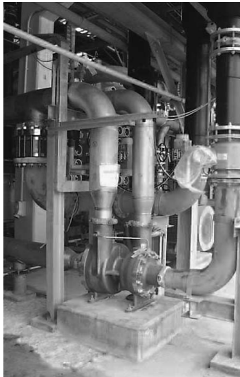
FIGURE 14.19 Turbocharger on 12,500 m 3 /day RO train.
