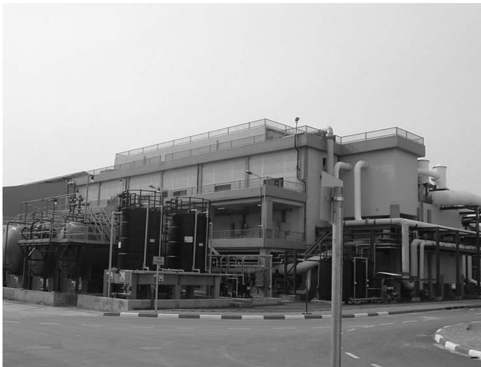
FIGURE 15.6 Calcite contactors of Ashkelon desalination plant, Israel.
