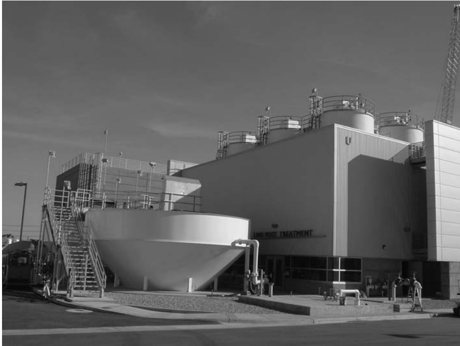
FIGURE 15.3 Lime storage silos and saturator.
