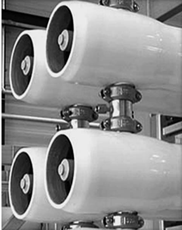
FIGURE 14.12 Multiple-port pressure vessels.
