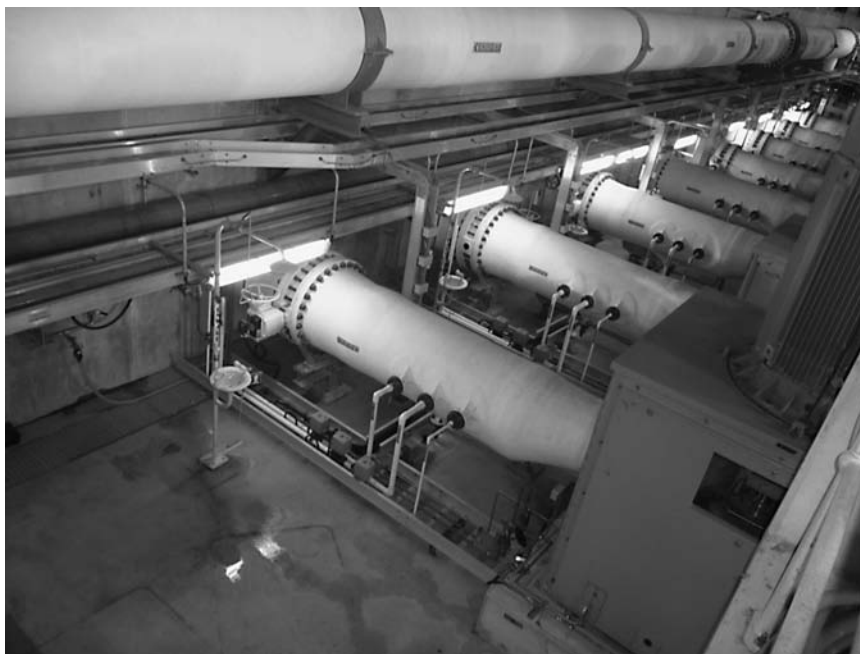
FIGURE 9.6 Point of chemical addition to pretreated water.
