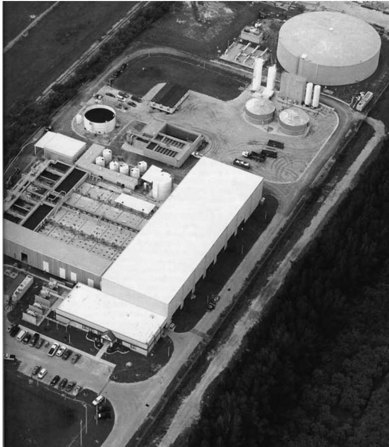
FIGURE 4.10 Layout of the Tampa Bay SWRO desalination plant, Florida. ( Tampa Bay Water. )
