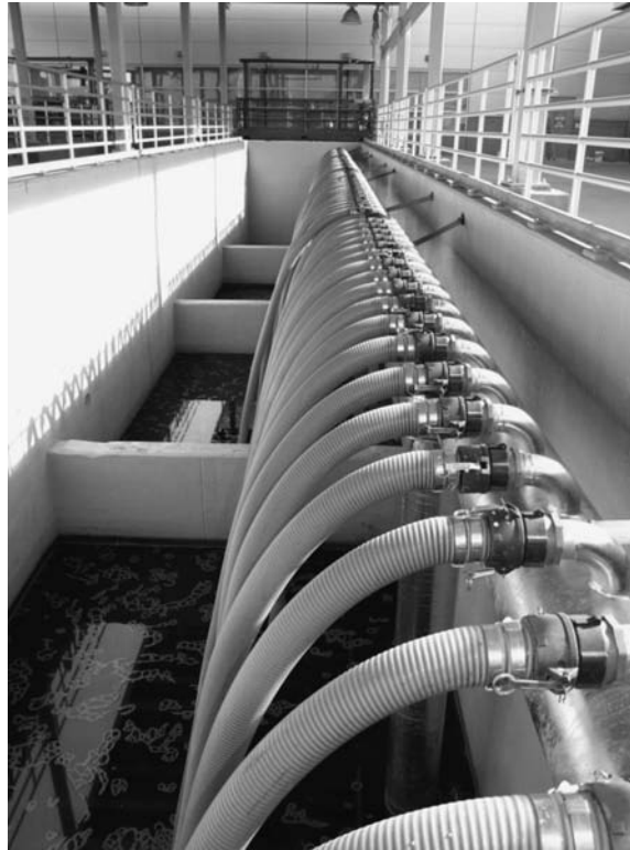
FIGURE 12.5 Submerged MF system.
