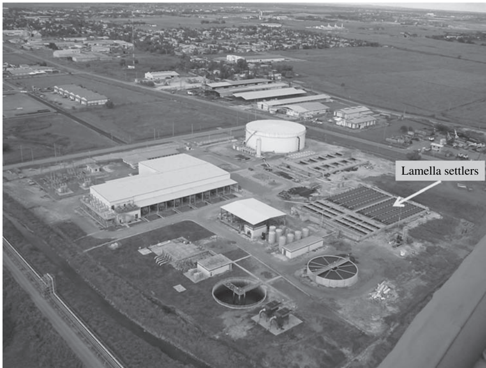
FIGURE 10.2 Point Lisas desalination plant, Trinidad. (Source: Desalcott.)
