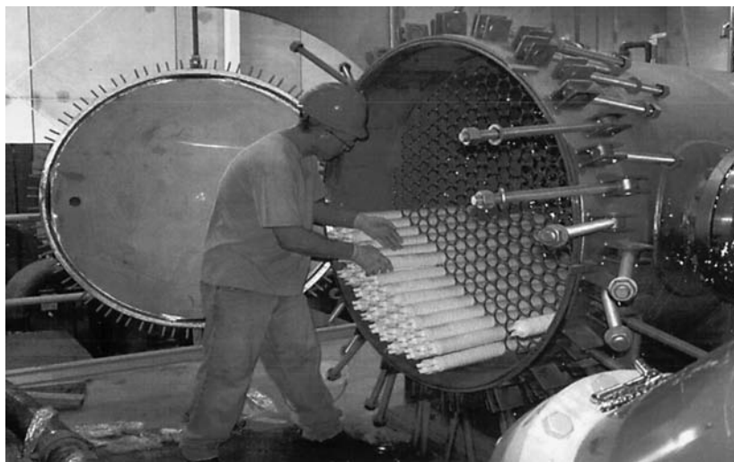
FIGURE 8.15 Cartridge filters installed in a horizontal vessel.
