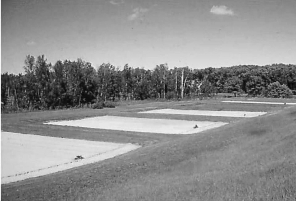
FIGURE 16.32 Rapid infiltration basins.
