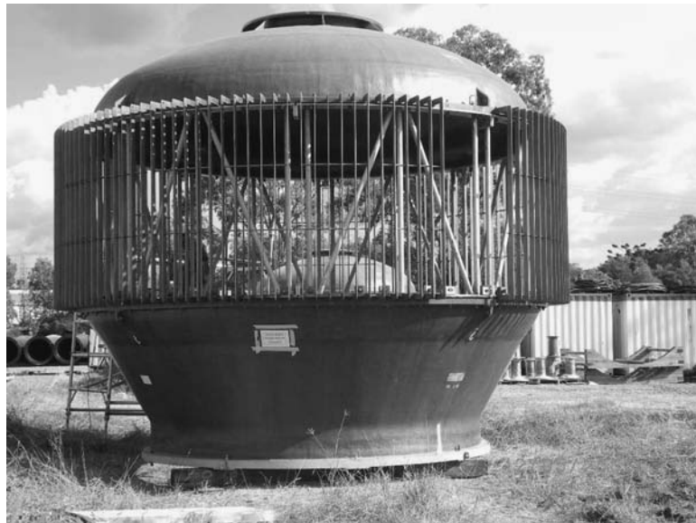
FIGURE 5.1 Intake bar screen. (Source: GHD.)
