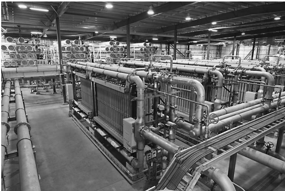
FIGURE 12.3 Pressurized MF system with vertical membrane elements.
