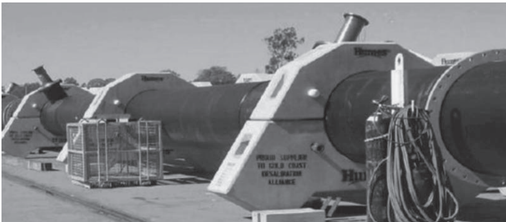
FIGURE 16.7 Gold Coast SWRO plant diffuser.
