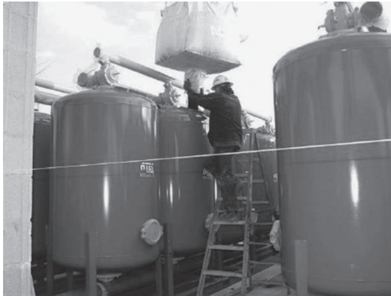
FIGURE 15.8 Refilling of calcite media.
