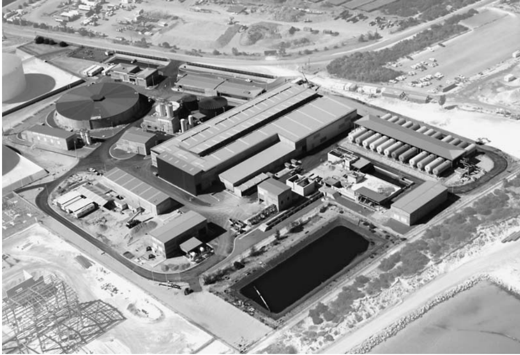
FIGURE 16.13 Perth seawater desalination plant. (Source: Water Corporation.)
