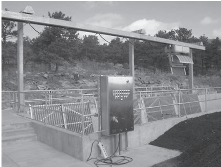
FIGURE 8.2 Coarse screen for onshore intake. (Source: Atlas.)
