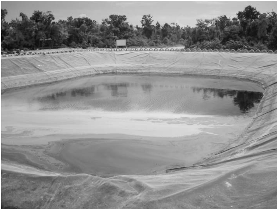
FIGURE 16.45 Geo-membrane evaporation pond liner.
