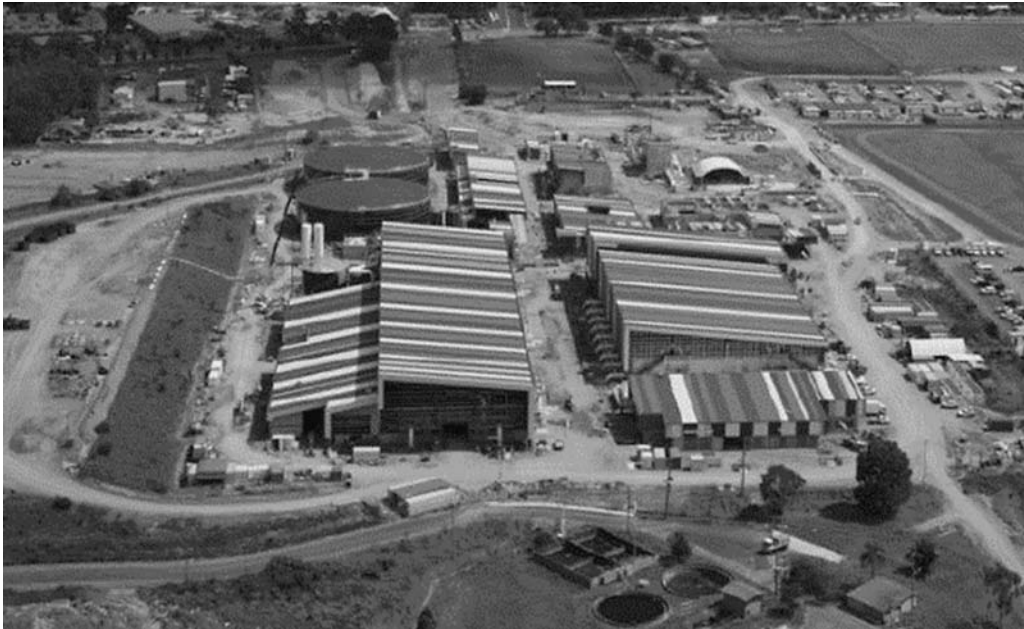
FIGURE 16.10 Gold Coast seawater desalination plant. (Source: Water Corporation.)
