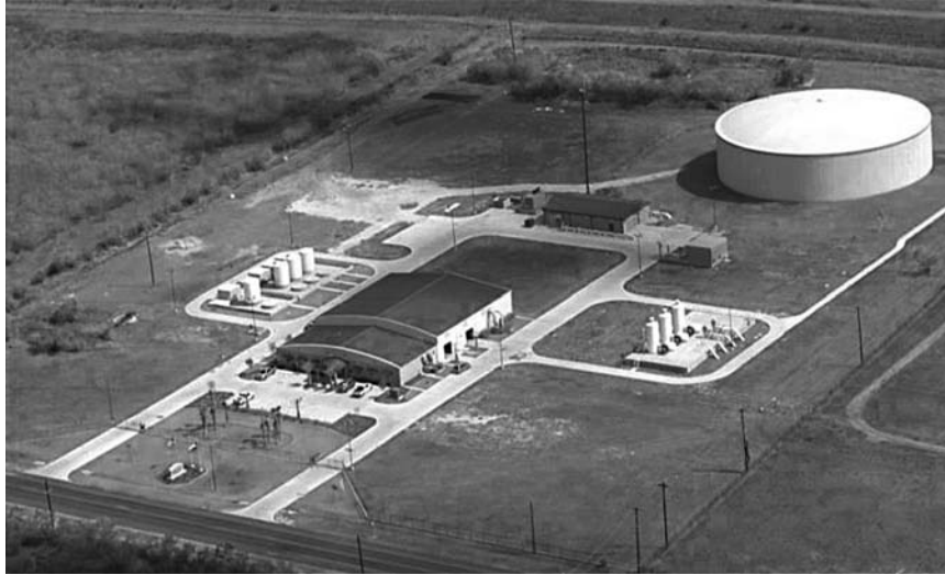
FIGURE 4.11 Layout of the Southmost BWRO plant, Brownsville, Texas. (Source: NRS Consulting Engineers.)
