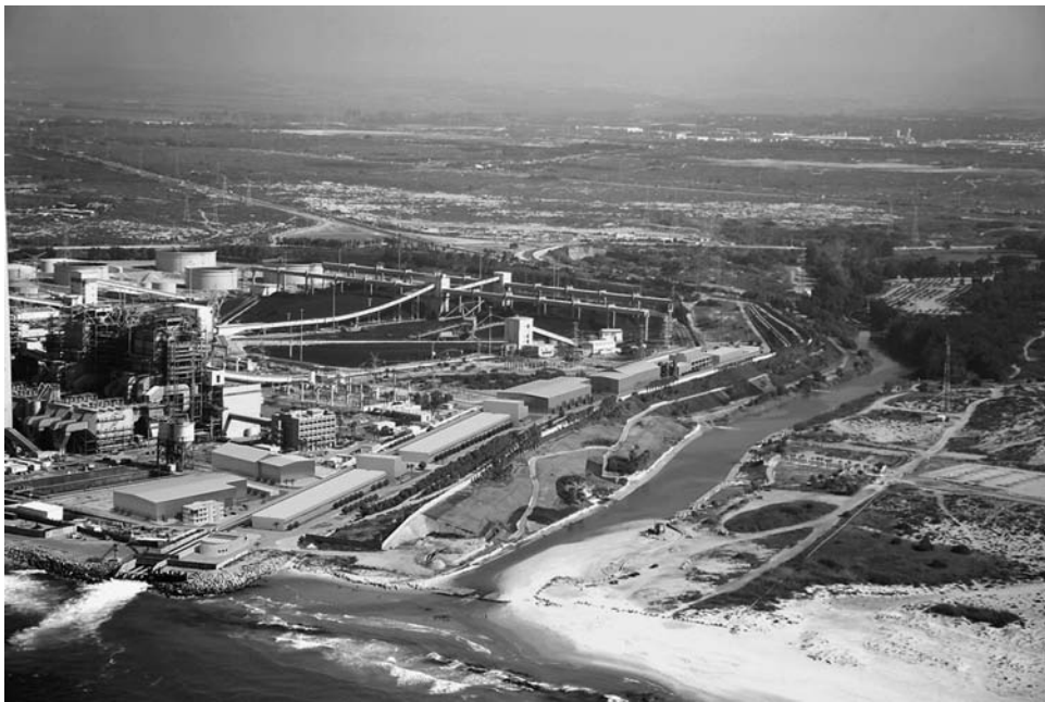
FIGURE 16.3 Near-shore discharge of Hadera SWRO Plant, Israel. (Source: IDE.)
