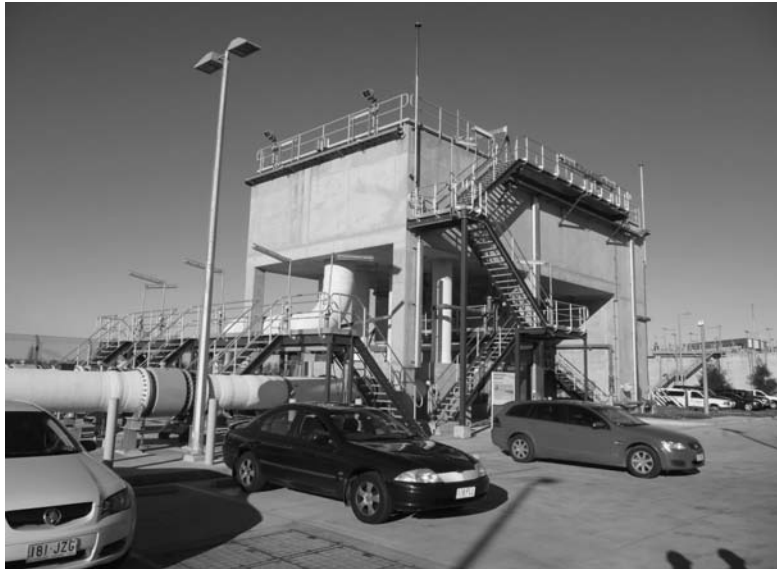
FIGURE 8.8 Drum screen intake structure of the Gold Coast Desalination Plant.
