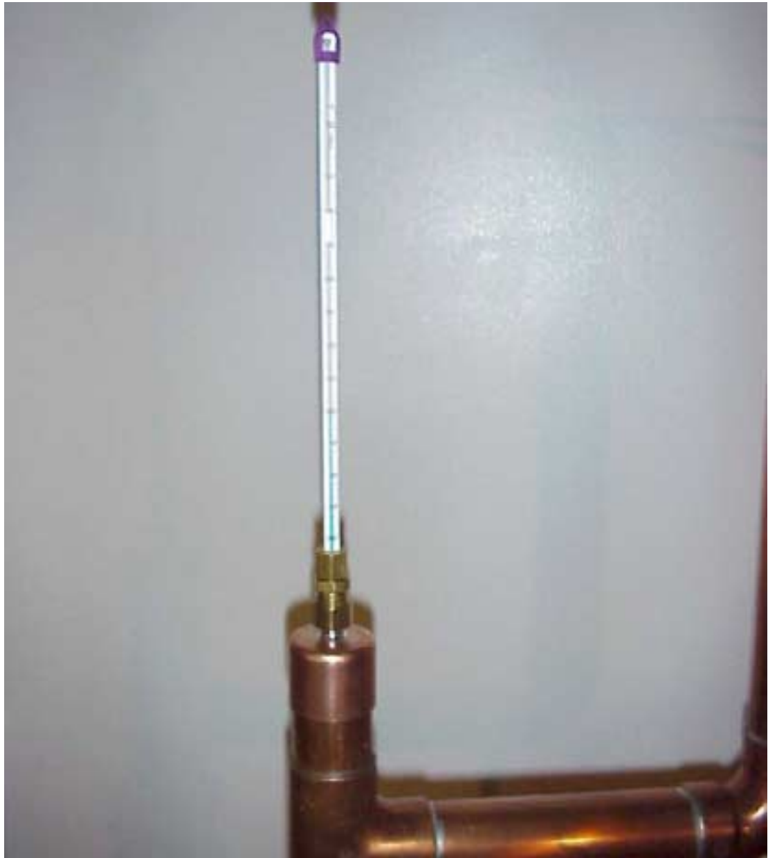
Thermometer Mounted with Compression Coupling
